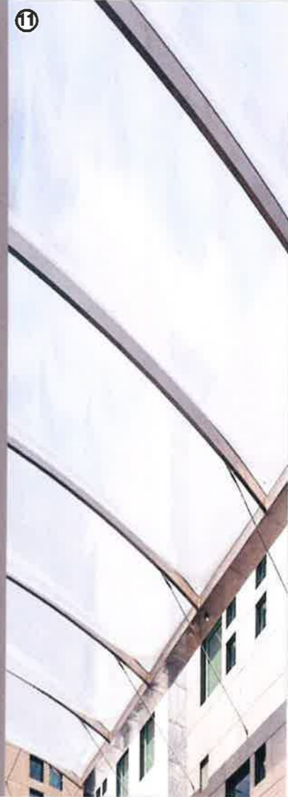
ETFE PILLOWS TO GRANDSTAND AND LEISURE POOL SHADE STRUCTURES
