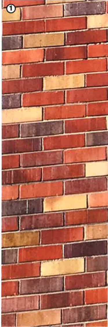
EXISTING BRICKWORKS TO EXISTING STAIR BUILDINGS
