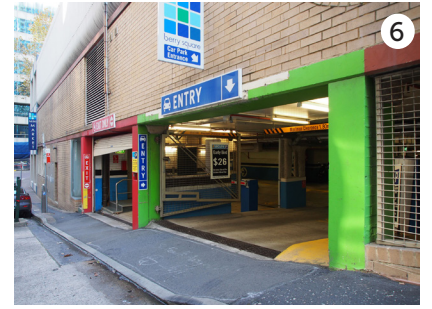
Vehicular entrance to Shopping World car park, Little Spring Street
