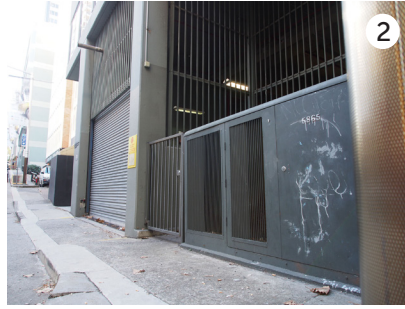
Rear of 88 Walker Street
