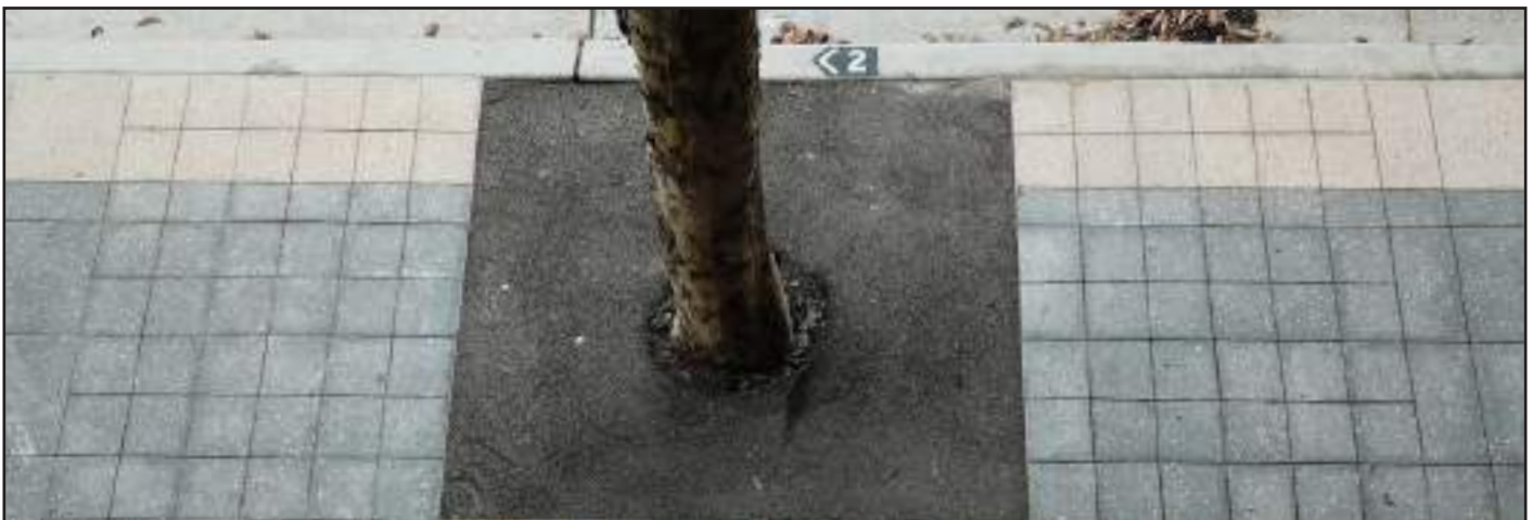
Recycled rubber surfacing to tree pit
