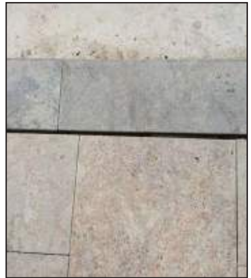
Existing Kerb treatment
