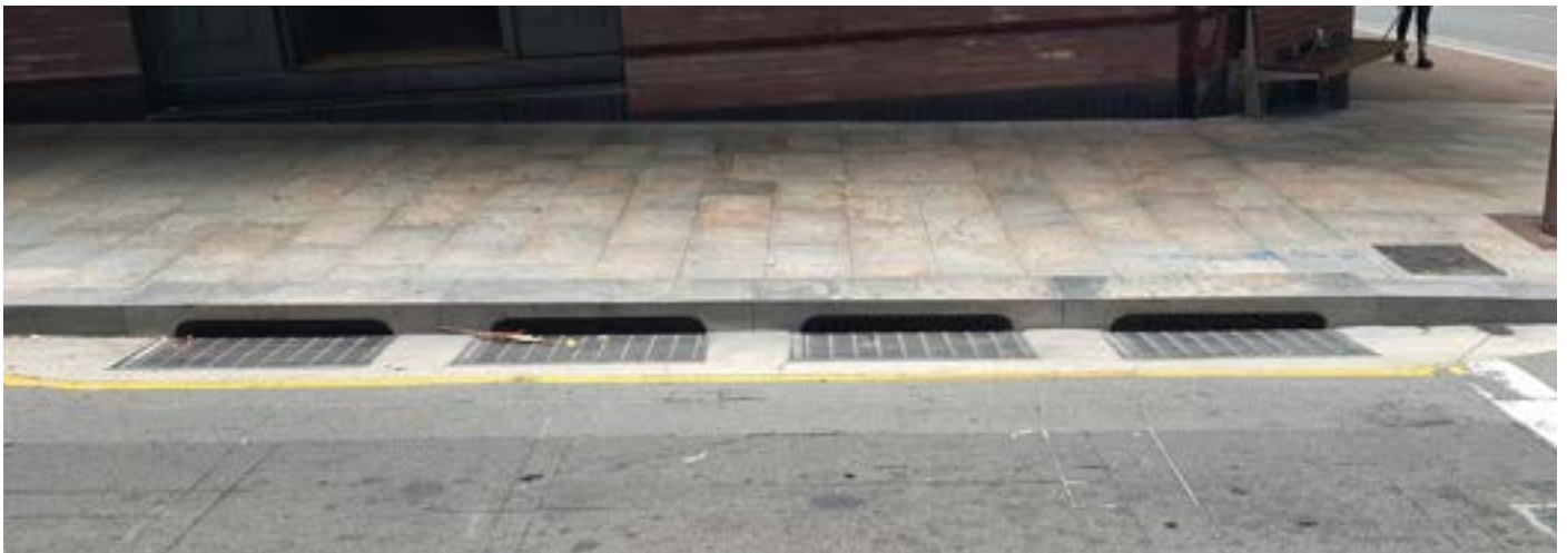
Typical Granite Stone Kerb and Concrete Gutter
