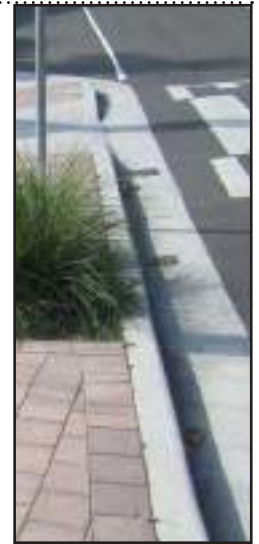
Shirley Road existing kerb and gutter treatment
