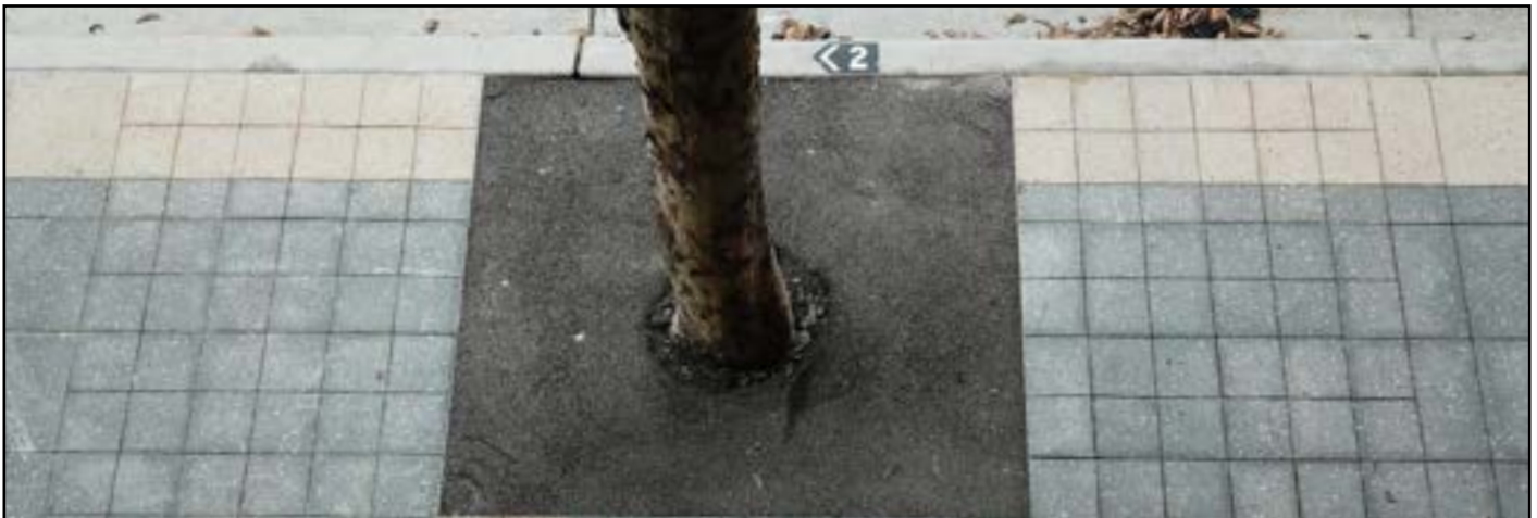
Recycled rubber surfacing to tree pit
