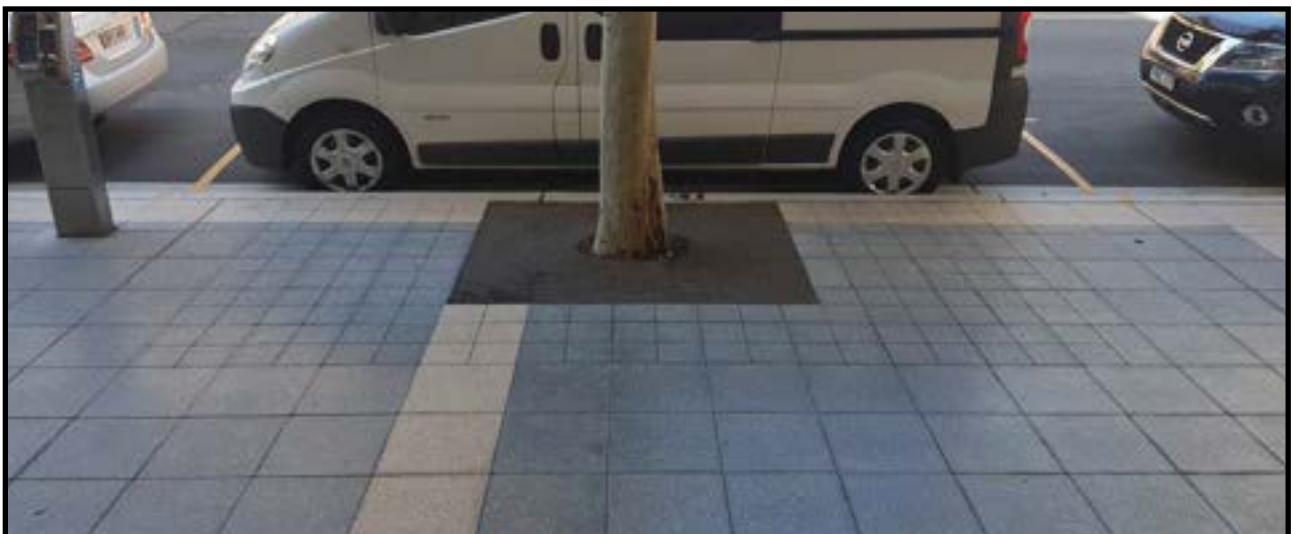
Recycled rubber surfacing to tree pit
