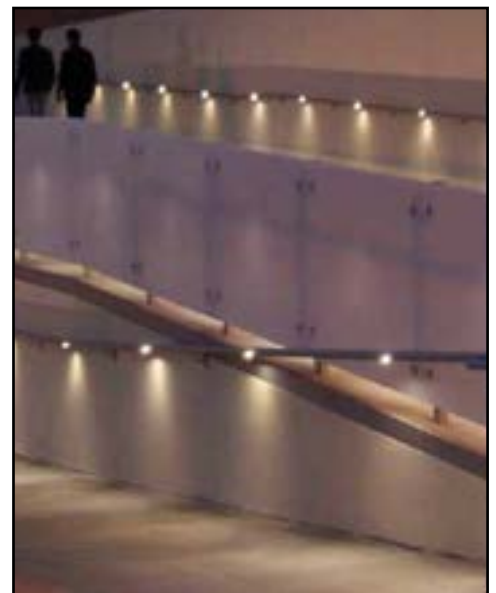
Indicative handrail lighting
