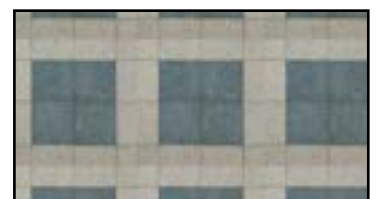
Precast concrete units in stackbond pattern
