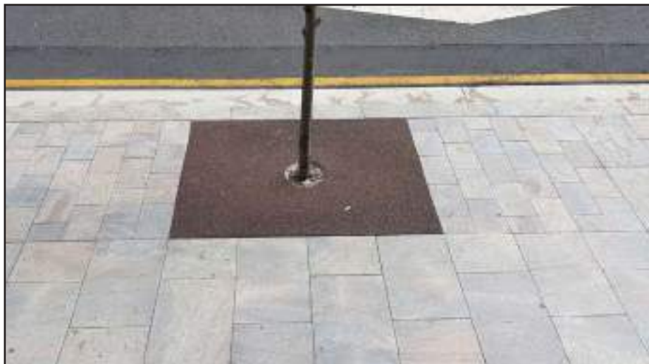
Porous rubber surfacing to tree pit
