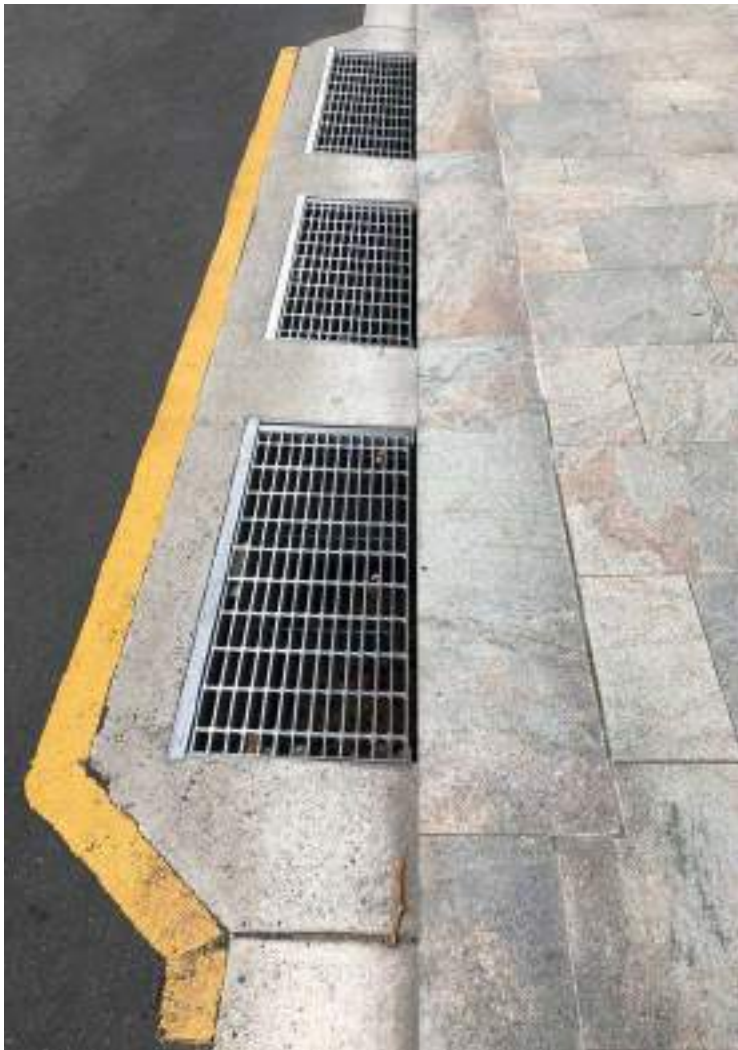
Typical Granite Stone Kerb and Concrete Gutter
