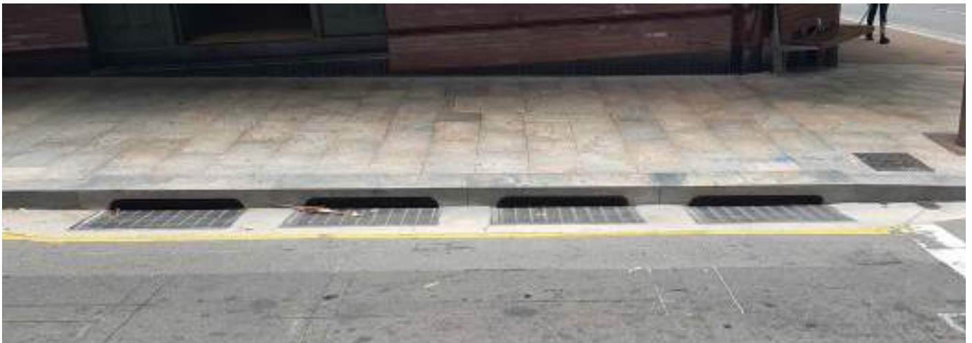
Typical Granite Stone Kerb and Concrete Gutter
