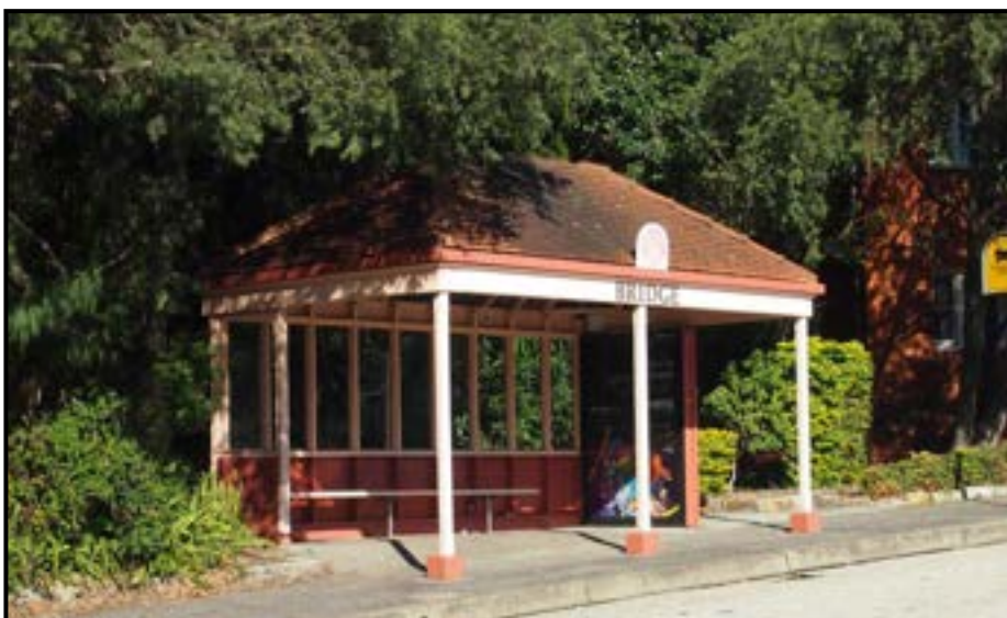
Existing bus stop - Cammeray
