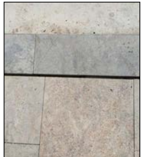
Existing Kerb treatment
