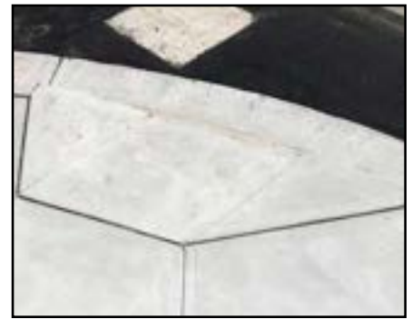
Existing kerb ramp in North Sydney Centre
