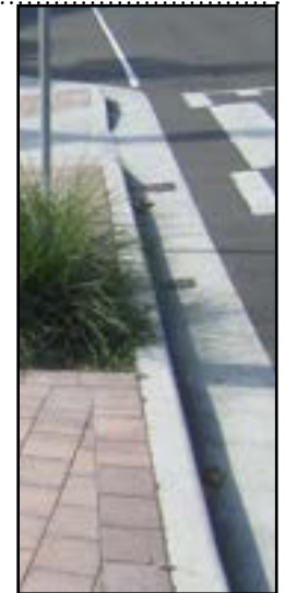
Shirley Road existing kerb and gutter treatment
