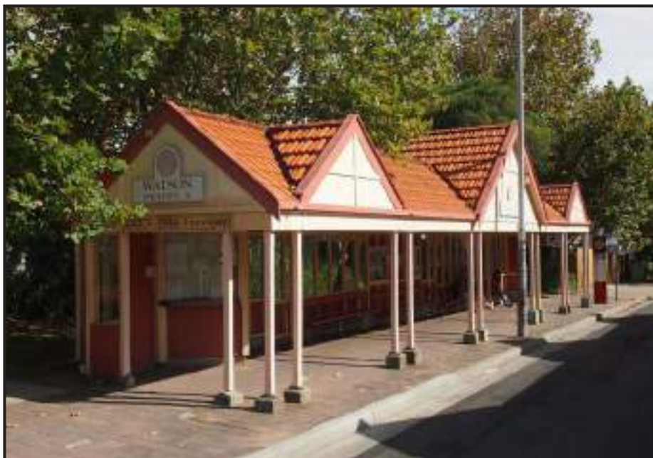
Existing bus stop - Neutral Bay
