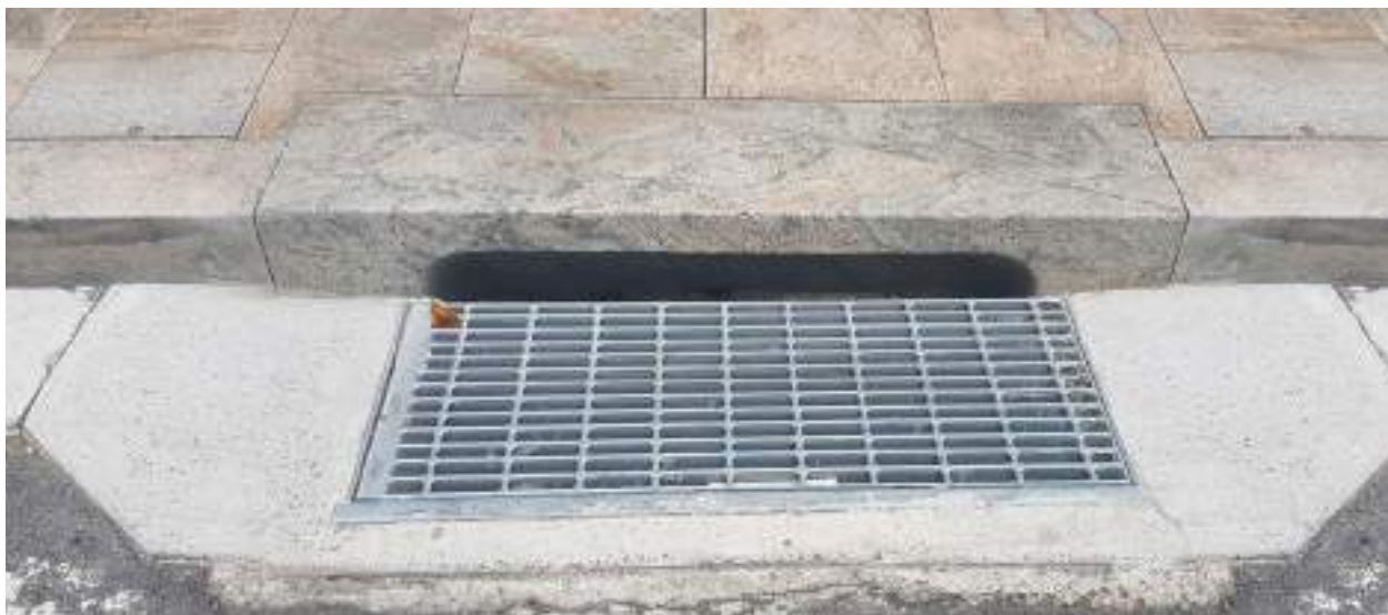
Typical Granite Stone Kerb and Concrete Gutter
