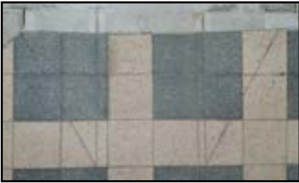
Existing kerb ramps in St Leonards
