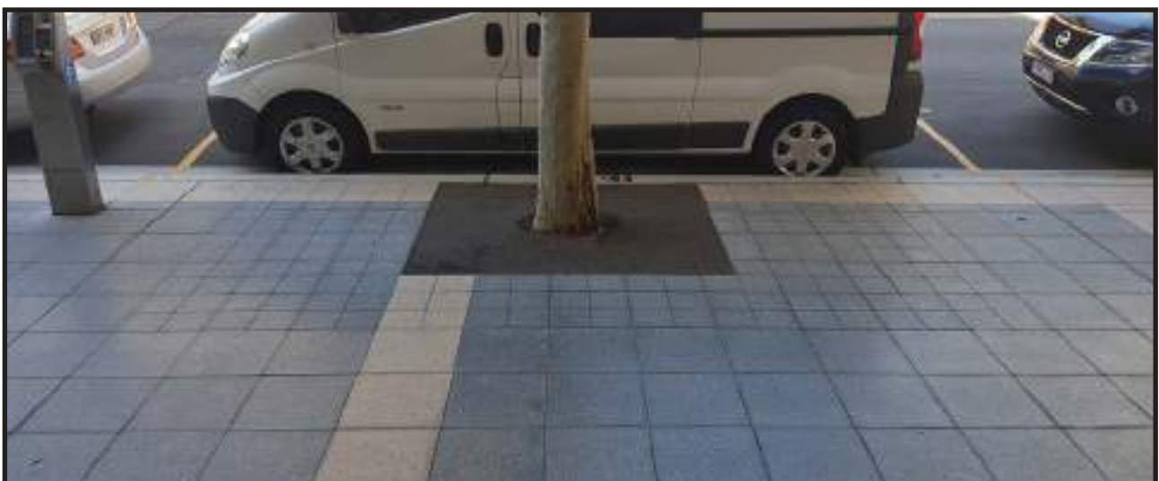
Recycled rubber surfacing to tree pit
