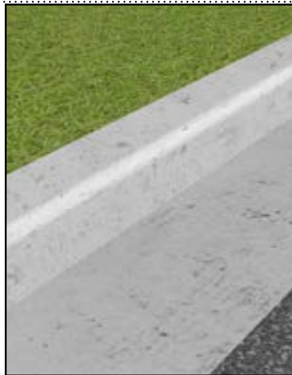
Kerb and gutter treatment
