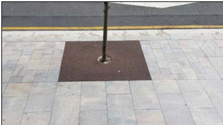
Porous rubber surfacing to tree pit
