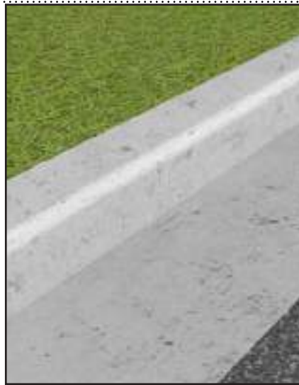
Kerb and gutter treatment
