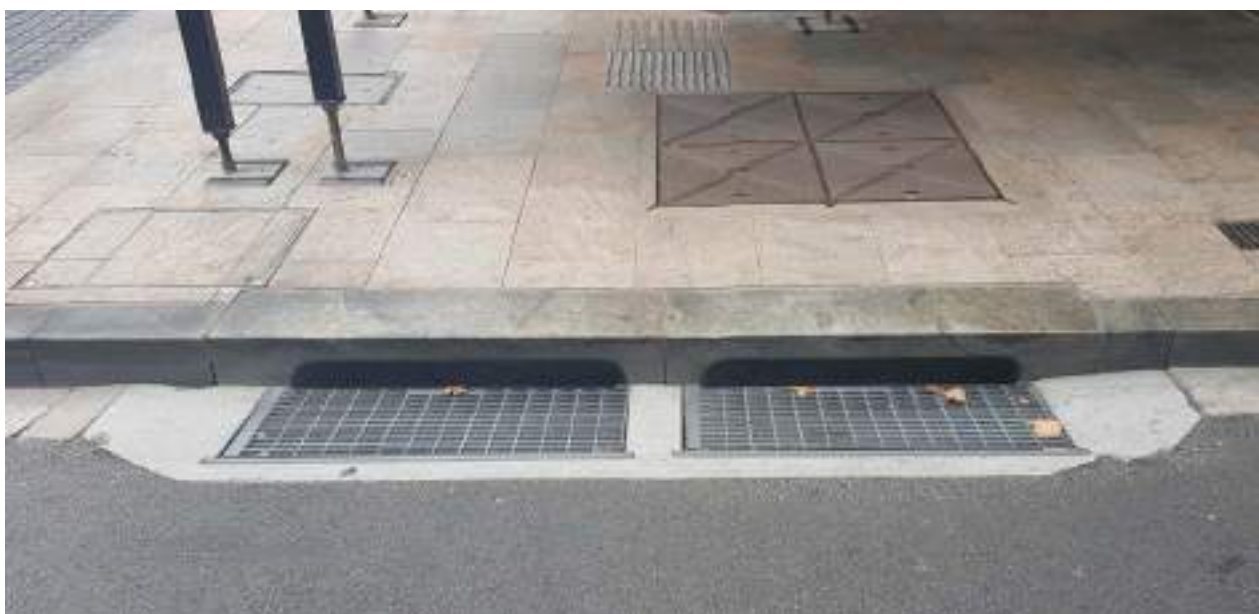
Typical Granite Stone Kerb and Concrete Gutter
