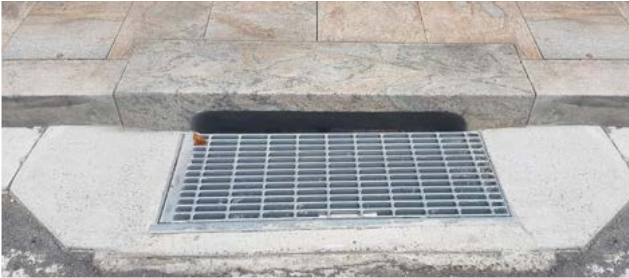
Typical Granite Stone Kerb and Concrete Gutter
