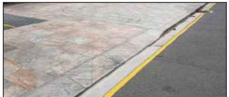
Granite layback on Berry Street
