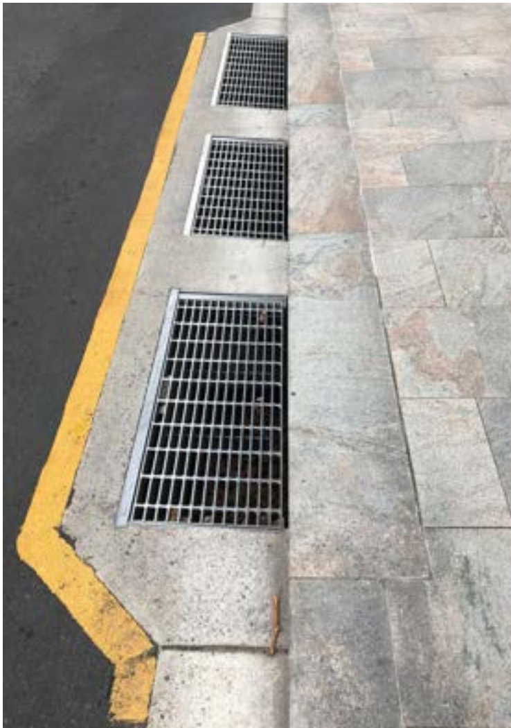
Typical Granite Stone Kerb and Concrete Gutter
