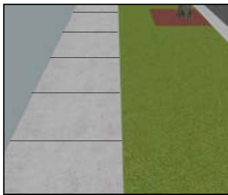
1.5m wide concrete footpath
