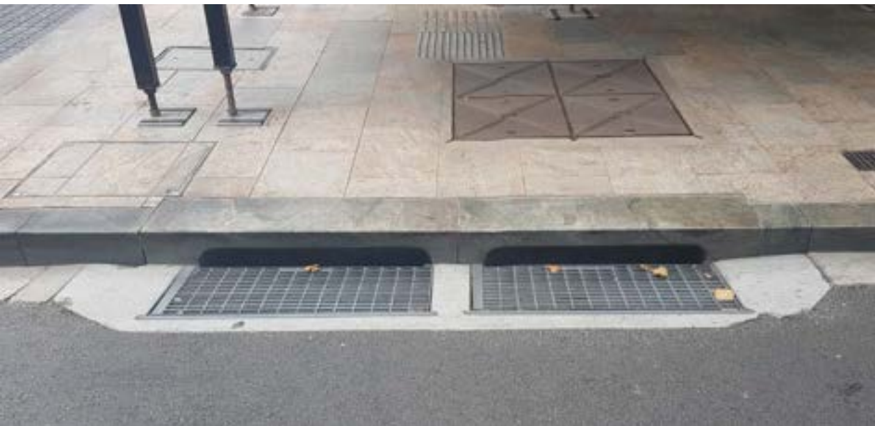
Typical Granite Stone Kerb and Concrete Gutter
