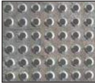
Stainless Steel Tactile Ground Surface Indicators
