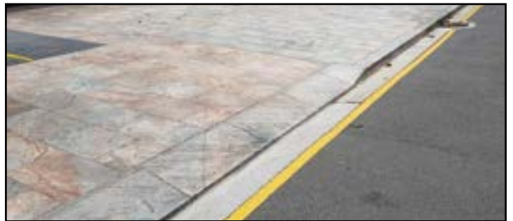
Granite layback on Berry Street
