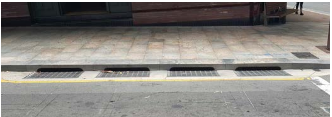
Typical Granite Stone Kerb and Concrete Gutter
