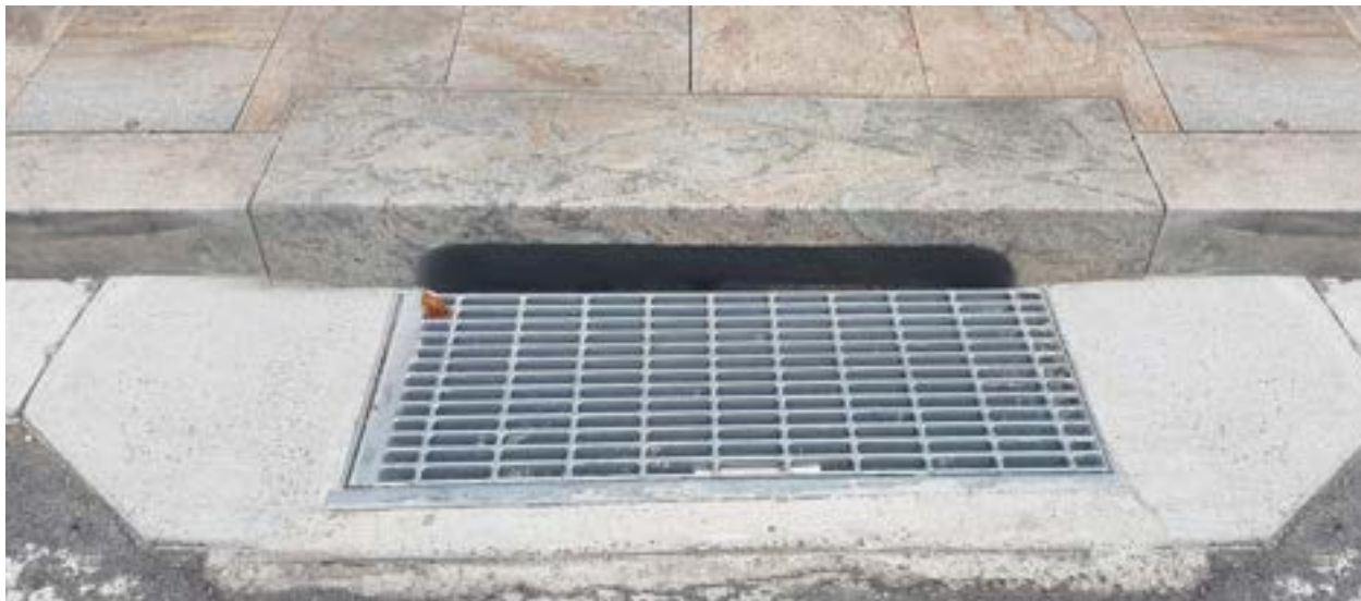
Typical Granite Stone Kerb and Concrete Gutter
