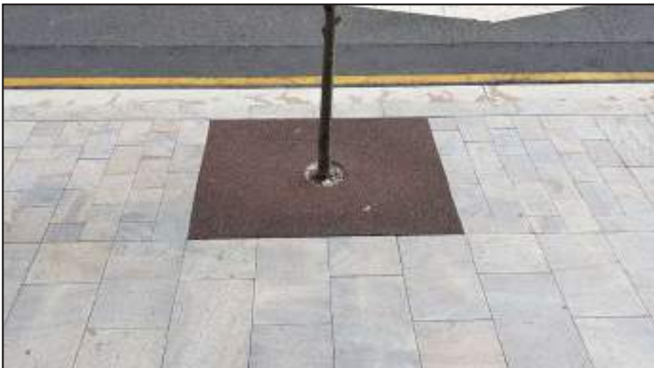
Porous rubber surfacing to tree pit
