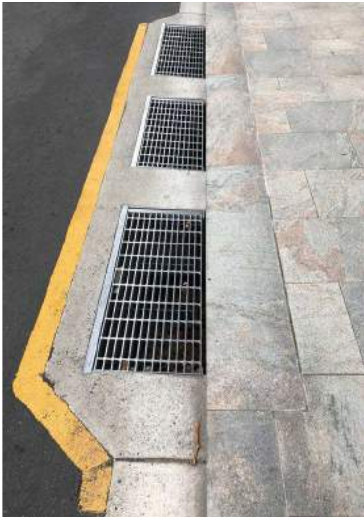
Typical Granite Stone Kerb and Concrete Gutter
