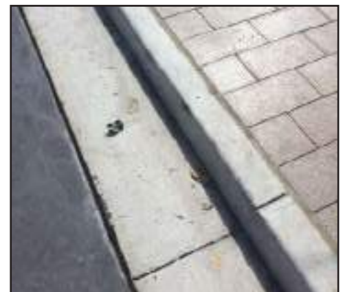
Existing kerb and gutter treatment
