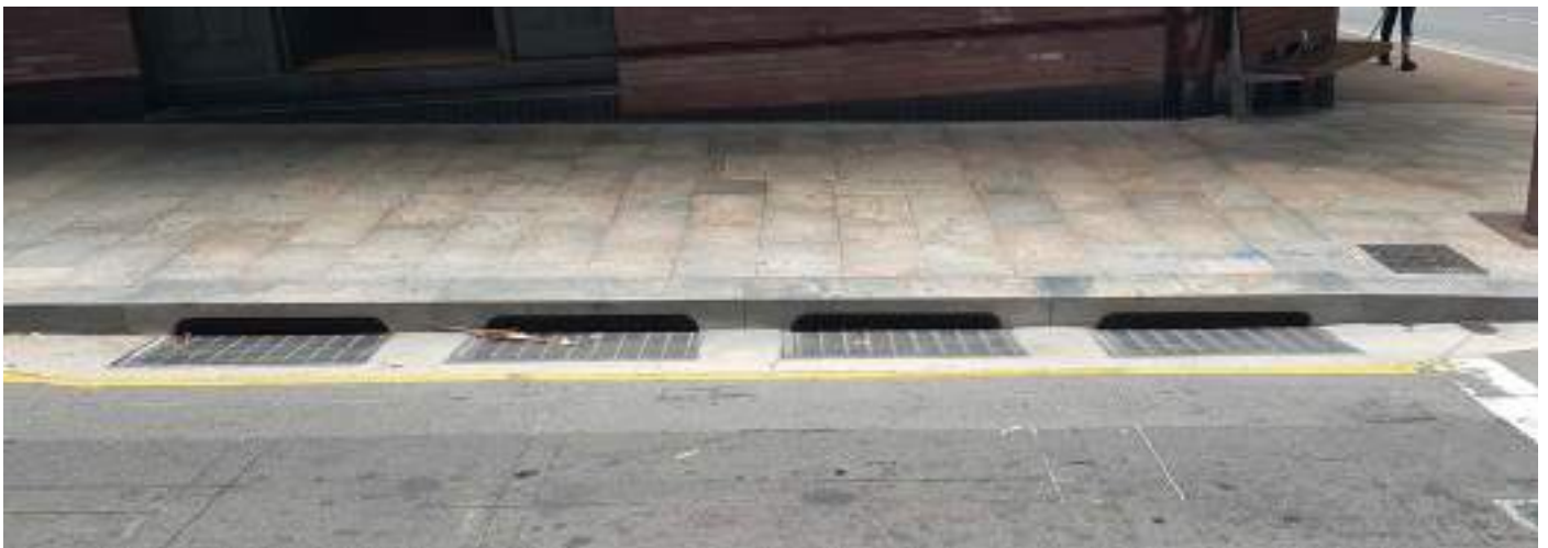
Typical Granite Stone Kerb and Concrete Gutter
