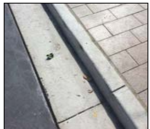
Existing kerb and gutter treatment
