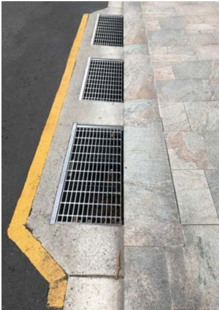
Typical Granite Stone Kerb and Concrete Gutter
