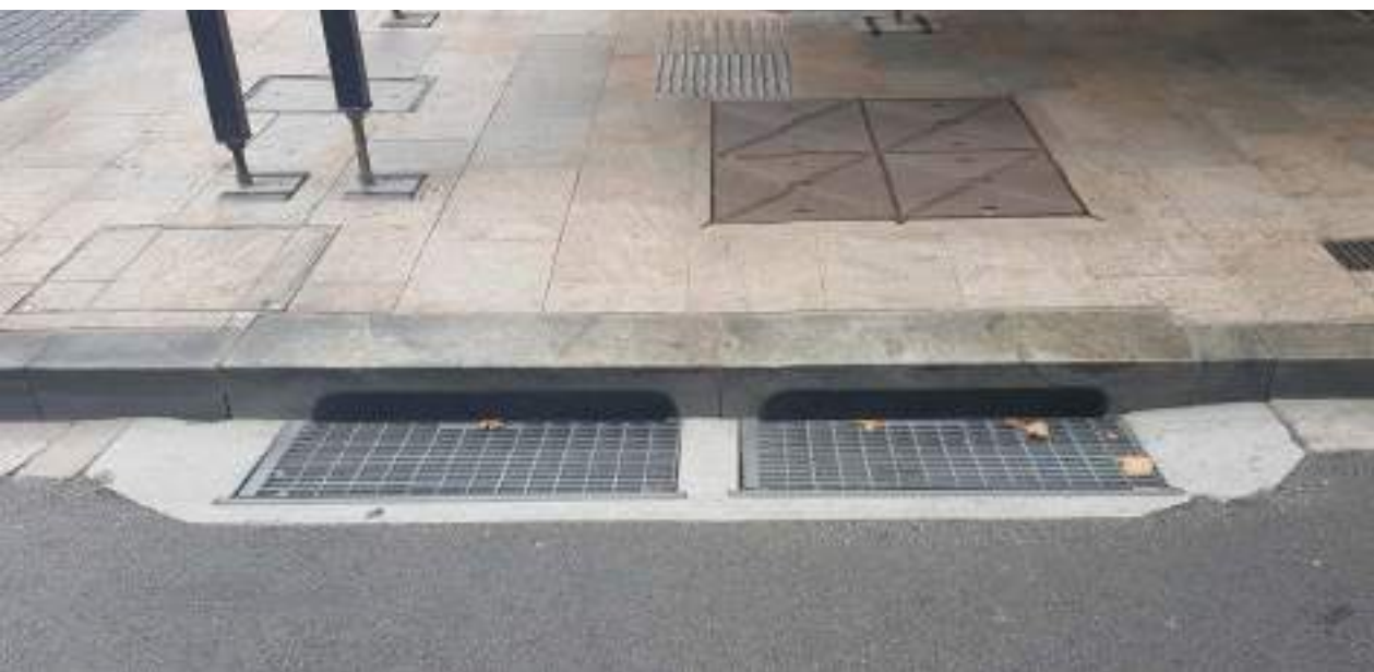
Typical Granite Stone Kerb and Concrete Gutter
