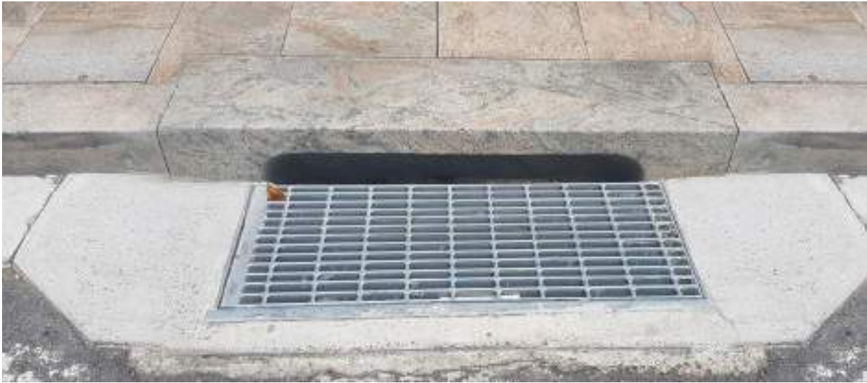
Typical Granite Stone Kerb and Concrete Gutter
