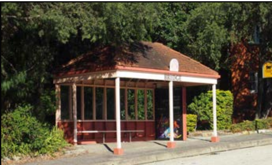
Existing bus stop - Cammeray
