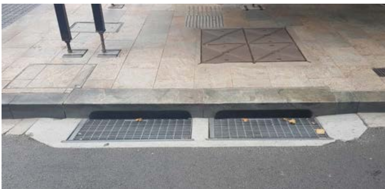
Typical Granite Stone Kerb and Concrete Gutter
