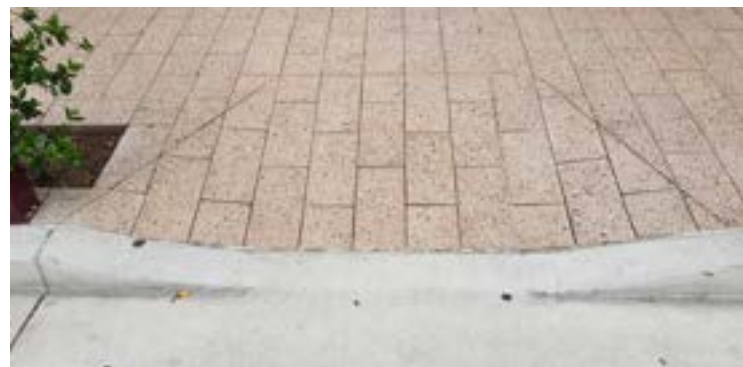
Typical kerb ramp
