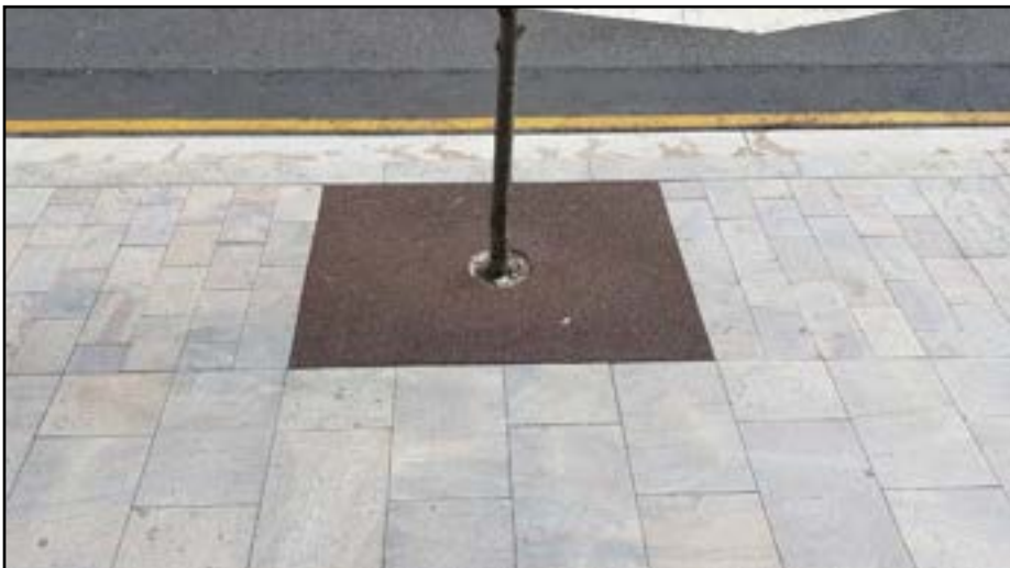
Porous rubber surfacing to tree pit
