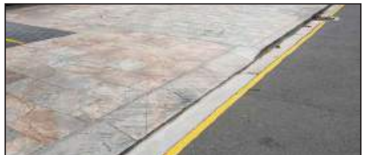
Granite layback on Berry Street
