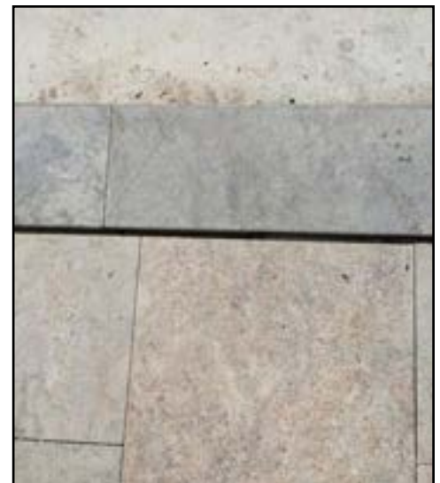
Existing Kerb treatment
