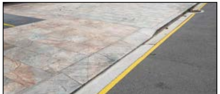
Granite layback on Berry Street
