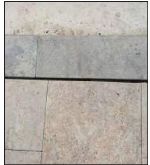
Existing Kerb treatment
