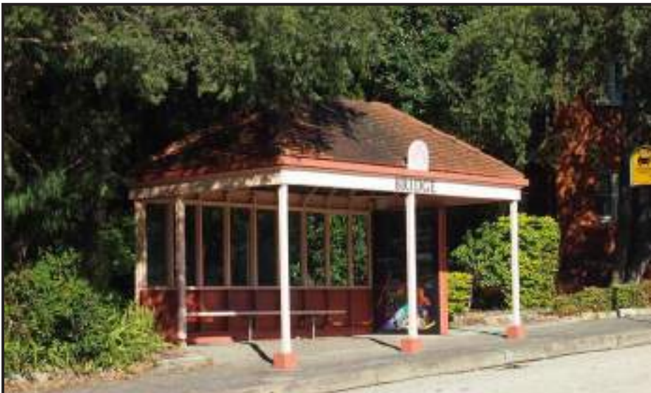
Existing bus stop - Cammeray
