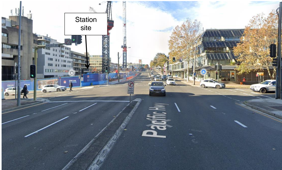
Figure 3 – Looking south along the Pacific Highway at the Oxley Street intersection.
