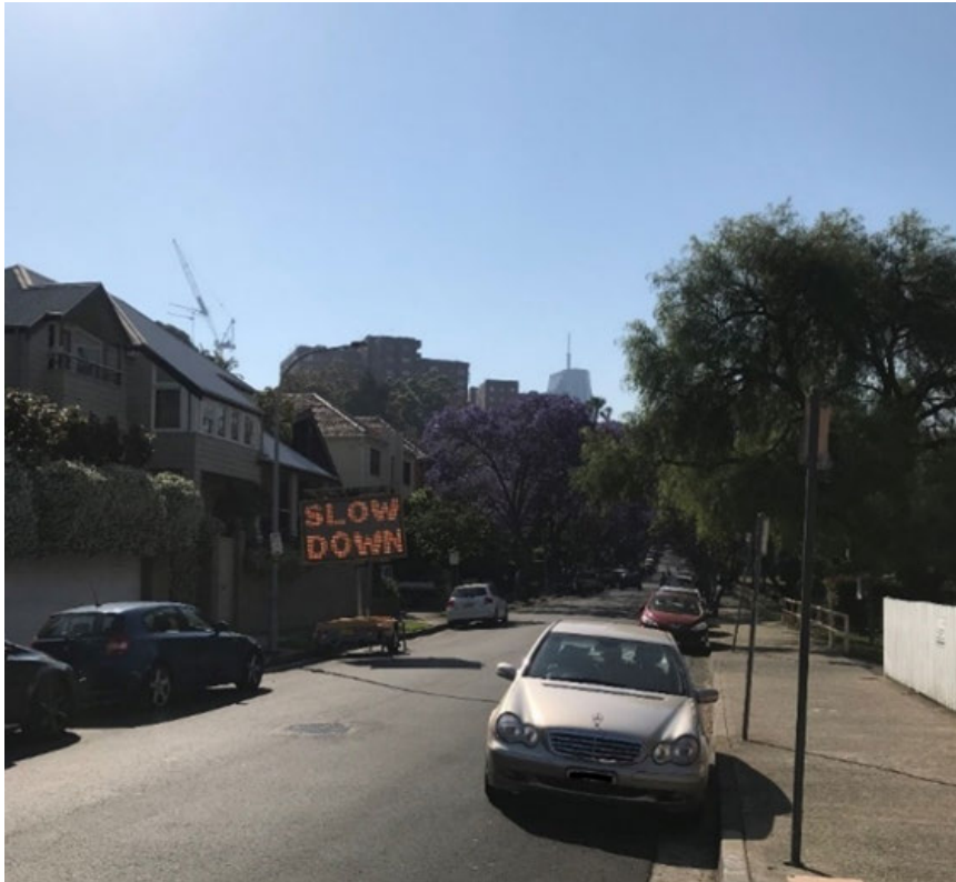
Photo 3. VMS Signs installed in McDougall Street during the 2019 Season
