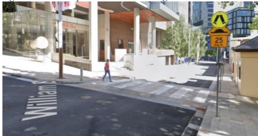
Figure 2 Raised pedestrian crossing William Street at Mount Street
