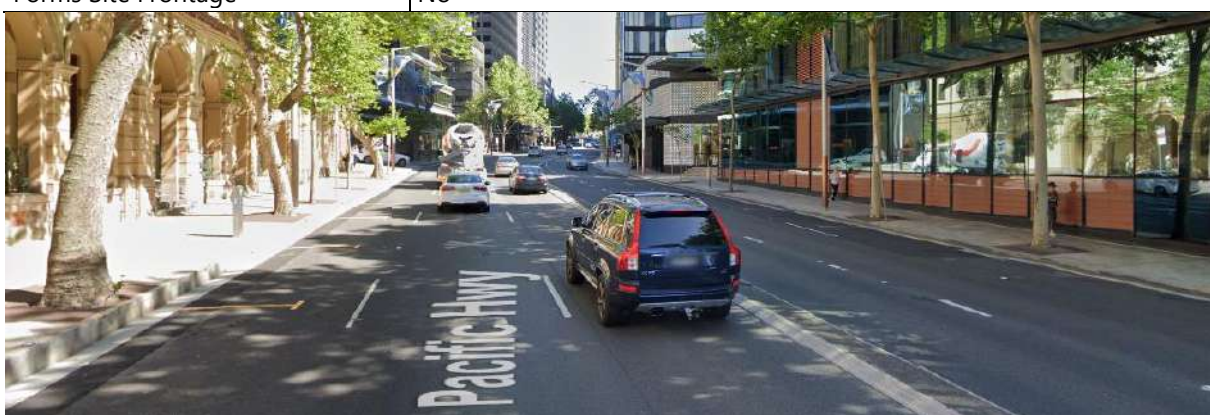
Figure 13 - Pacific Highway (Northbound)
