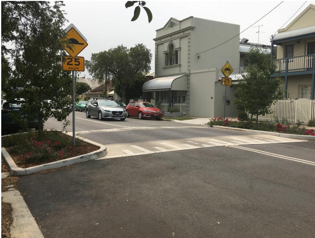
Figure 1. Example flat top threshold (note – where there is existing on-street parking, garden beds are omitted to preserve parking)
