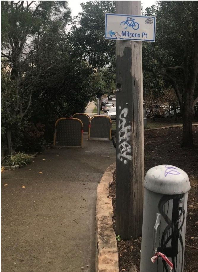
Figure 3 Existing chicanes in St Peters Park
