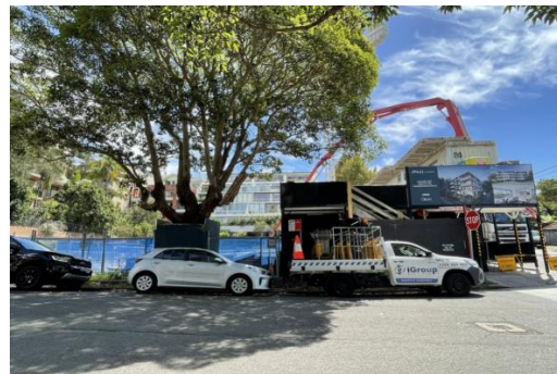
Figure 4.29 View of a lot currently under construction, representative of the development of the area.
