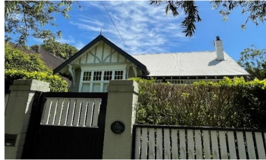
Figure 4.10 View showing a detail of the roof form, with decorative timber detailing, brackets and finial.
