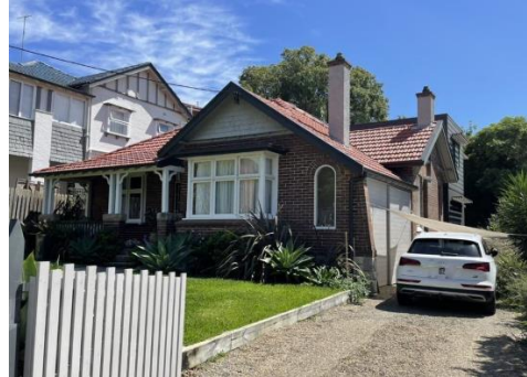
Figure 4.15 View showing the eastern elevation, roof form and temporary car shade, looking northwest.
