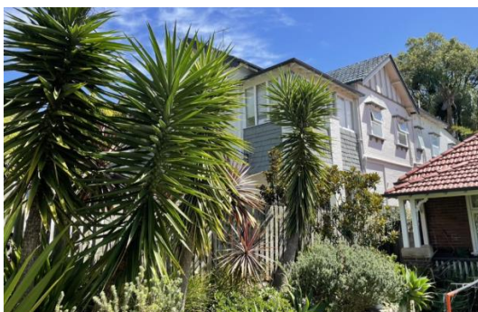
Figure 4.18 View showing a detail of the upper storey of the eastern elevation. The enclosed balcony, with timber detailing, is visible.
