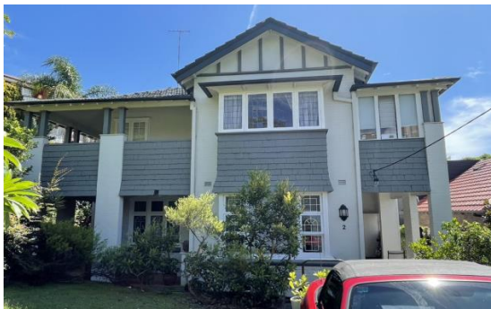
Figure 4.16 View of the primary elevation of 125 Holt Avenue, looking north.
