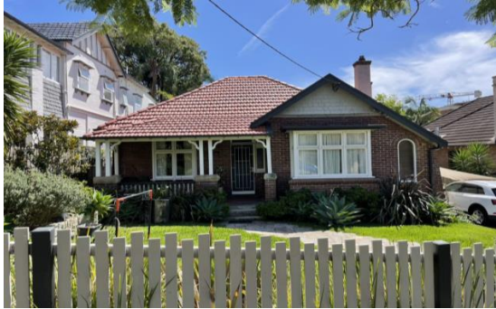
Figure 4.14 View showing the primary elevation of 123 Holt Avenue, looking north.
