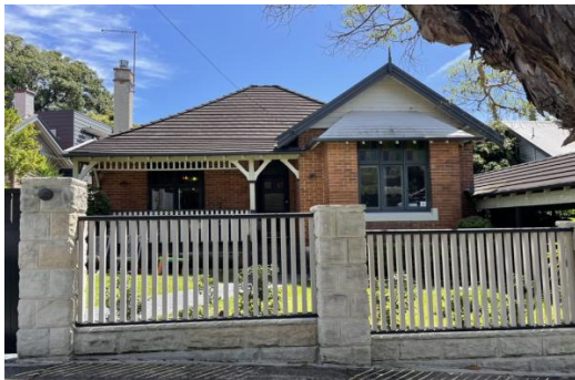
Figure 4.11 View of the primary elevation of 121 Holt Avenue, looking north.
