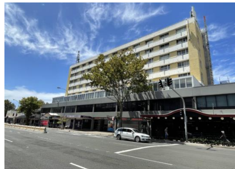
Figure 4.25 View of mixed use commercial buildings along Military Road, which would form the northwestern boundary of the proposed HCA.
