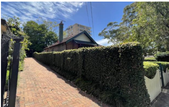
Figure 4.3 View of the western elevation and the original chimney, looking northeast.
