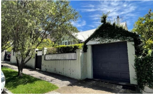
Figure 4.9 View showing the garage addition, looking northwest.
