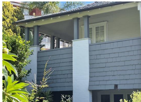
Figure 4.17 Detailed view of the balcony with rendered columns with timber accent, and timber shingles, looking northwest.
