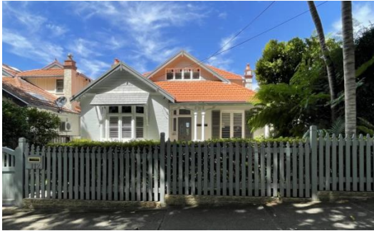
Figure 4.34 View of a typical Federation dwelling with a modified attic space.
