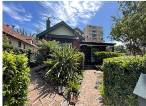
Figure 4.2 View showing the verandah and access path.
