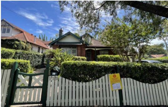
Figure 4.1 View of the property at 115 Holt Avenue, looking north.
