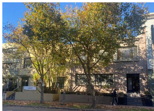
FIGURE 5: View of subject site along Chandos Street.
