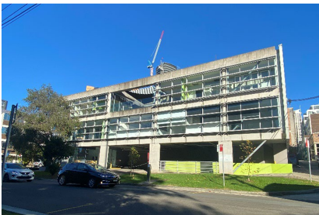
Figure 9 Existing development south of the site at 58-64 Atchison Street
