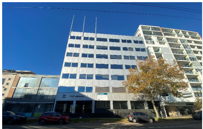
Figure 10 Existing development west of the site at 55-69 Chandos Street
