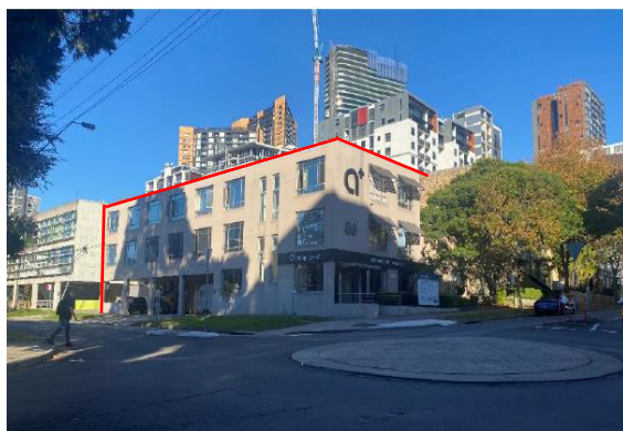
FIGURE 4: View of subject site from corner Oxley Street and Chandos Street.
