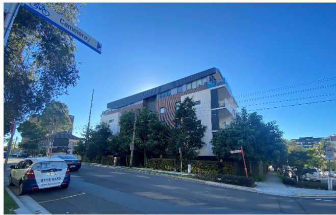
Figure 8 Existing development east of the site along Oxley Street
