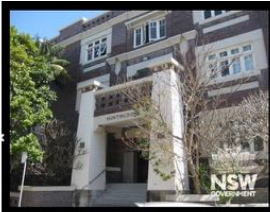
6 Holbrook Avenue, Kirribilli Source: Heritage NSW SHI form
