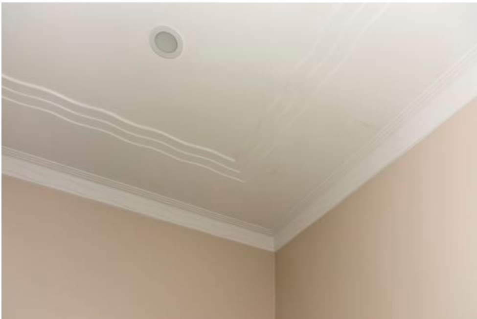
Figure 33: Original cornice detail to Unit 1 bedroom
