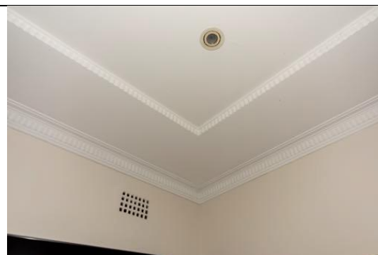
FIGURE 12: Original cornice to Unit 3 living room ceiling.
