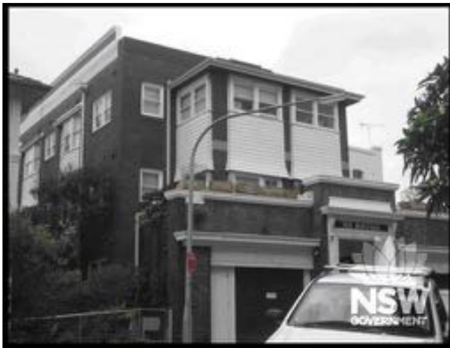
21 Holbrook Avenue, Kirribilli Source: Heritage NSW SHI form
