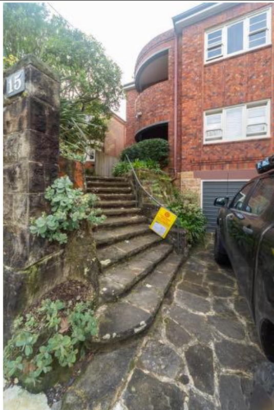
FIGURE 6: View from entry area showing tapestry brick panels to the façade and (at left) curved balconies with brick balustrades.
