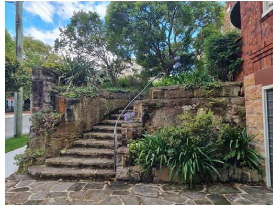
FIGURE 5: Sandstone entry steps at the site.
