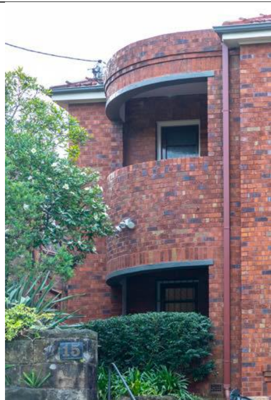
FIGURE 6: Curved corner balconies.
