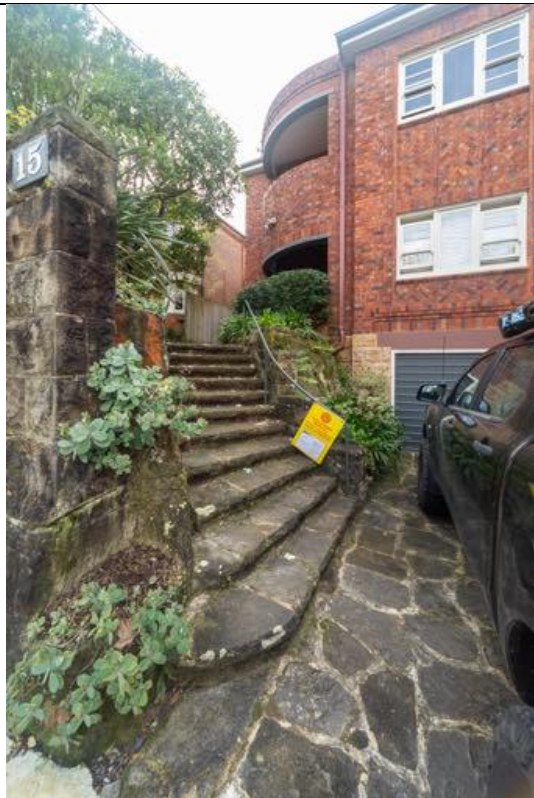
FIGURE 5: View from entry area showing tapestry brick panels to the façade and (at left) curved balconies with brick balustrades.
