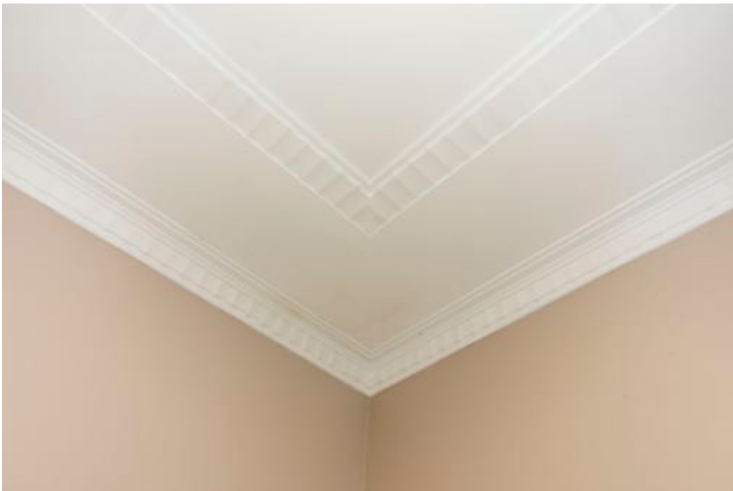
Figure 35: Cornice detail to 2 nd bedroom ceiling, Unit 1
