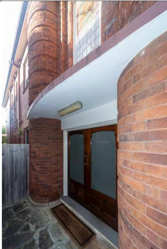
FIGURE 7: Detail around main entry doors.
