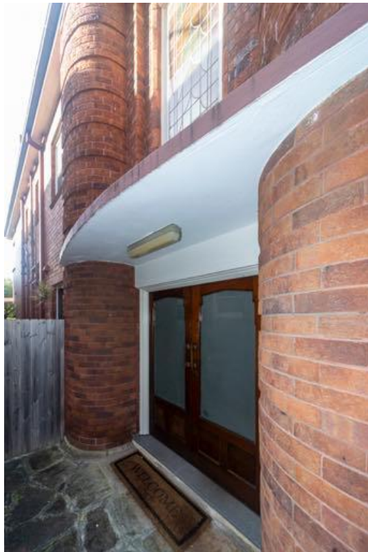
FIGURE 8: Detail around main entry doors.
