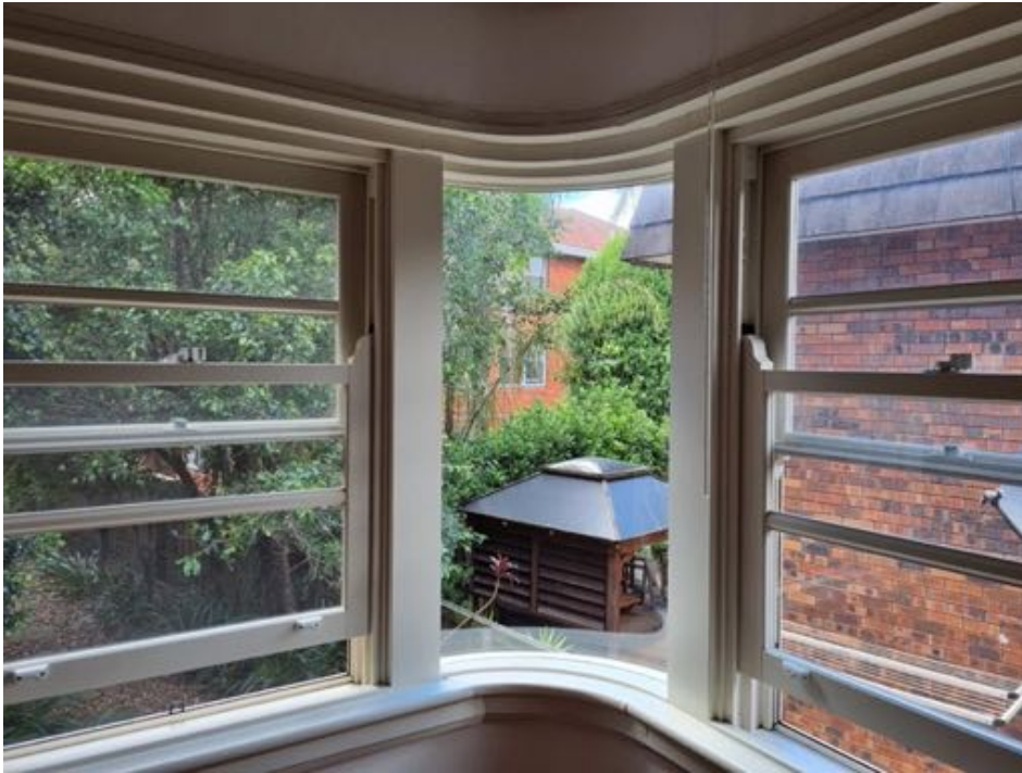
Figure 24: Curved glass to corner, with typical timber framed double hung windows with horizontal glazing bars to either side. Source: photo supplied by North Sydney Council
