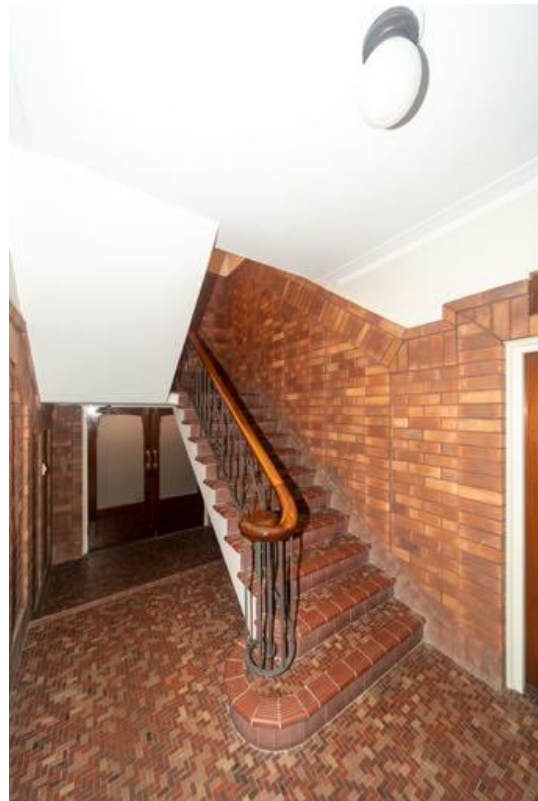
FIGURE 9: Original stairway in lobby showing original staircase, original tiling and brick and plaster wall finish.
