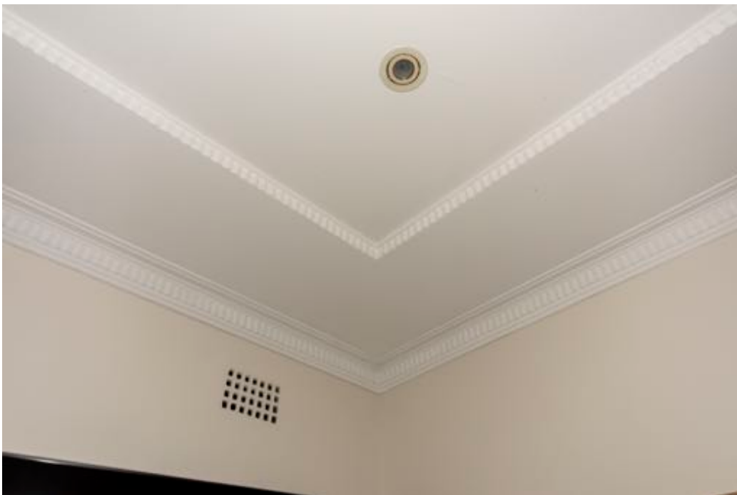
Figure 43: Original cornice to Unit 3 living room ceiling
