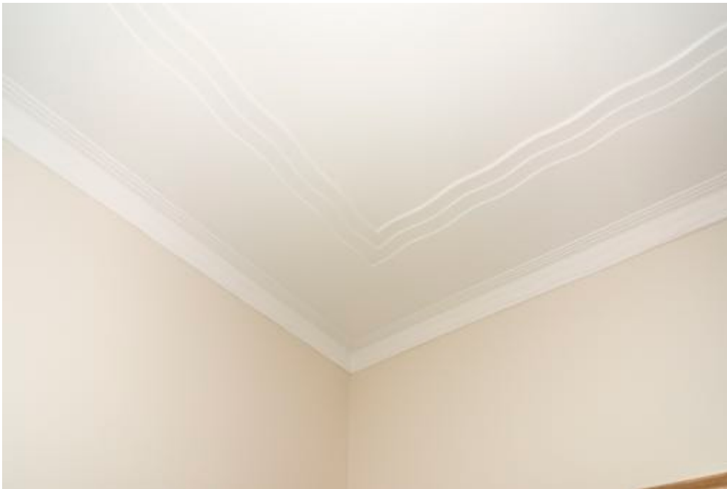
Figure 49: Unit 3 cornice detail to 2 nd bedroom
