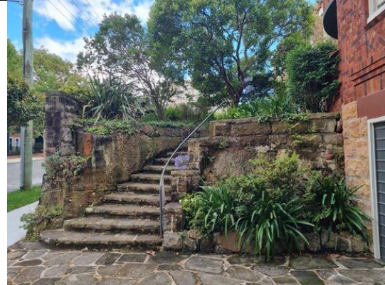
FIGURE 4: Sandstone entry steps at the site.
