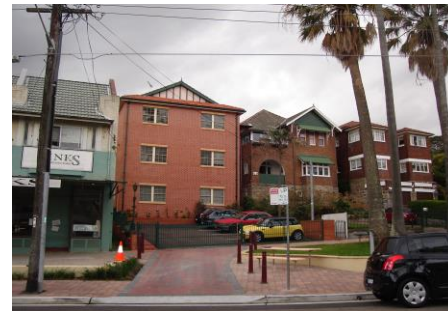
Figure B-13.17: Poor infill development does not respond well to adjoining characteristic developments.
