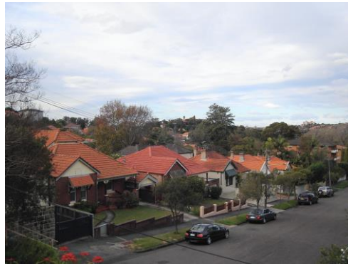
Figure B-13.13: Buildings from the nineteenth and early twentieth centuries often have steep pitches and formal geometry that combines to give a distinctive skyline.
