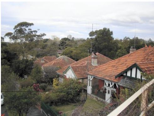
Figure B-13.12: Roofs can be unifying elements of conservation areas.
