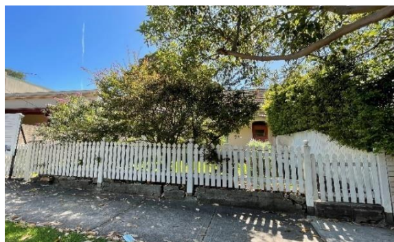
Figure 5.69 View of the primary elevation of 133 Holt Avenue, looking northeast.
