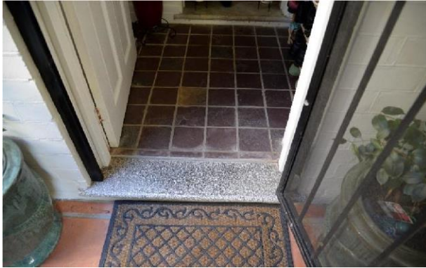
Figure 5.52 First floor apartment to west— terrazzo threshold.
