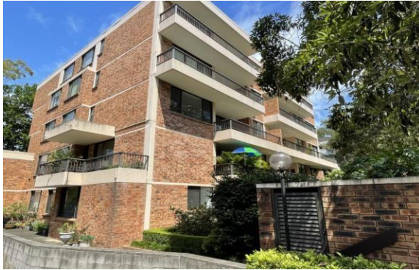
Figure 4.28 View of a typical contemporary apartment building.
