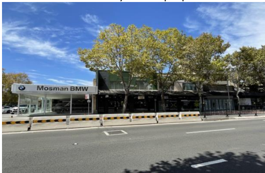
Figure 4.26 Typical view of commercial properties and lots along Military Road.
