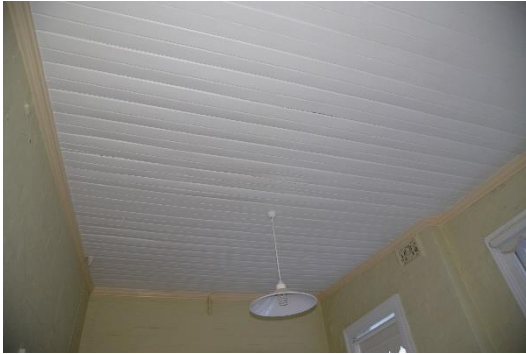
Figure 5.77 View of the original timber ceiling to the rear.
