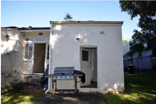
Figure 5.78 View of the rear façade of 133 Holt Avenue.
