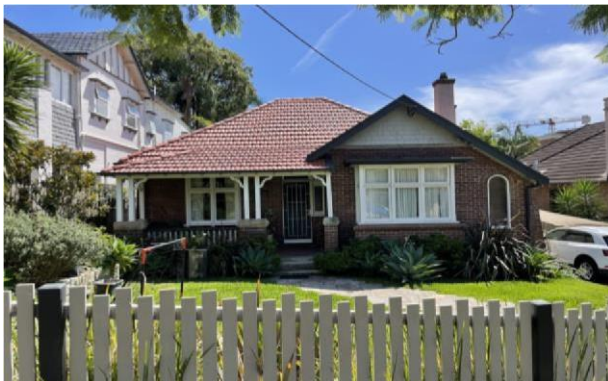
Figure 5.42 View showing the primary elevation of the eastern side of 123 Holt Avenue, looking north.
