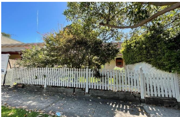
Figure 4.21 View of the primary elevation of 133 Holt Avenue, looking north-east.
