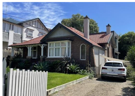
Figure 4.15 View showing the eastern elevation, roof form and temporary car shade, looking northwest.
