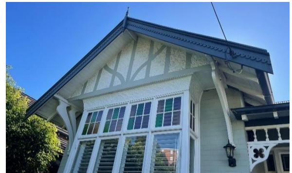
Figure 5.32 View showing a detail of the gable end, with decorative half-timbering, roughcast finish, timber brackets and bargeboards and finial and pressed metal cladding.
