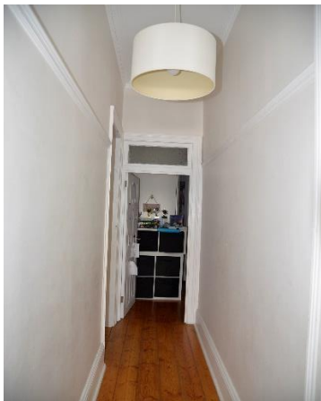
Figure 5.59 View of the central hallway.
