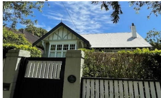
Figure 4.10 View showing a detail of the roof form, with decorative timber detailing, brackets and finial.
