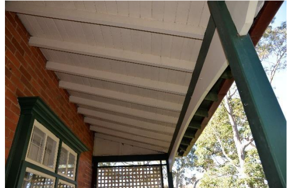
Figure 5.6 Timber ceiling, rafters and verandah.
