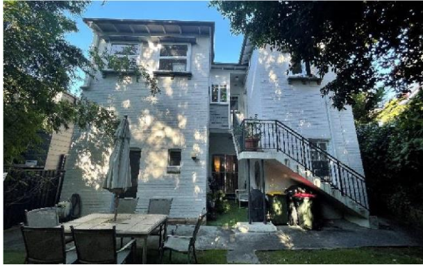
Figure 5.46 View of the rear elevation, facing south-west.
