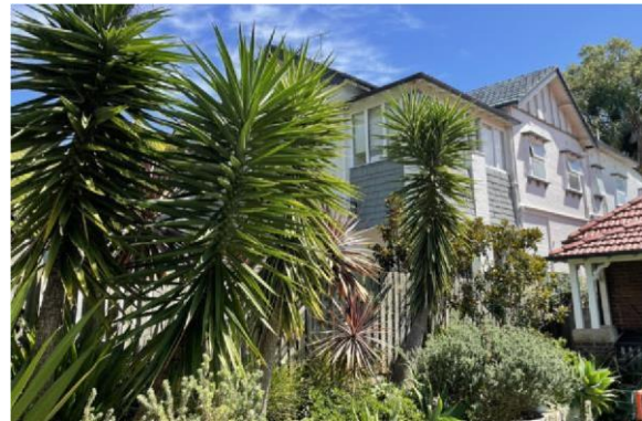
Figure 5.45 View showing a detail of the upper storey of the eastern elevation. The enclosed balcony, with timber detailing, is visible.
