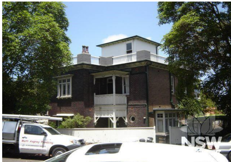
Figure 6.12 15–17 Bertha Road, Cremorne 'House'. (Source: NSW State Heritage Inventory)
