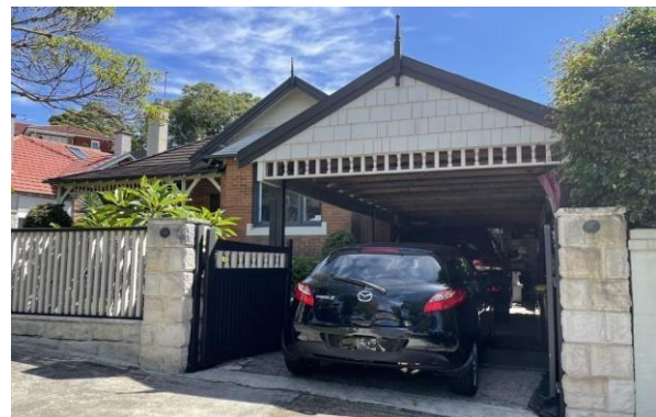
Figure 5.40 View showing the carport with matching timber shingles, looking northwest.
