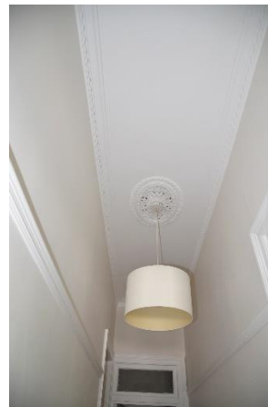
Figure 5.60 View of the ceiling to the central hallway.
