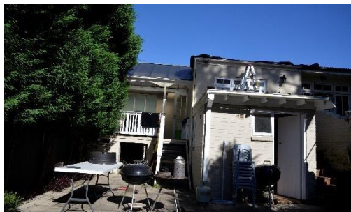
Figure 5.67 View of the rear elevation of 131 Holt Avenue.
