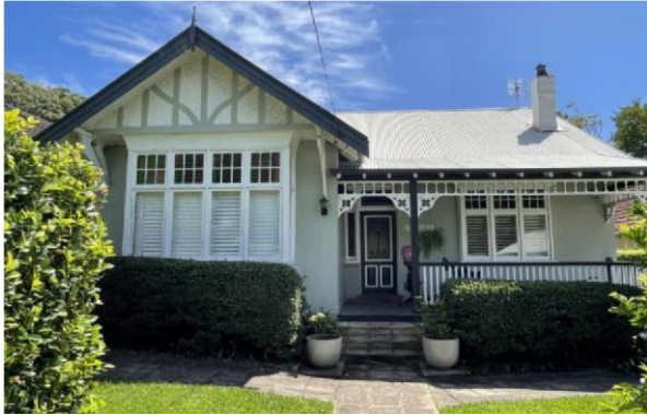
Figure 5.29 View of the primary elevation of 119 Holt Avenue.
