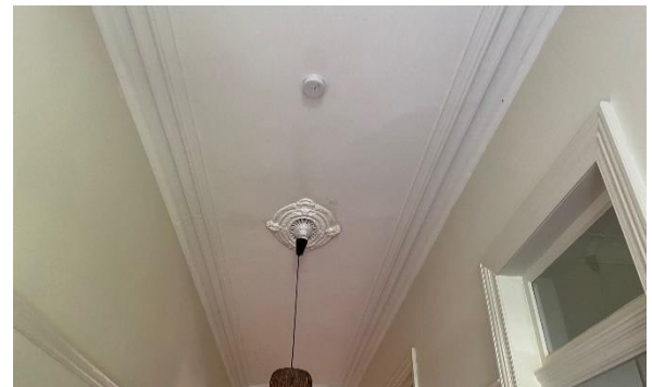
Figure 5.34 View of the ceiling rose along the central hallway.
