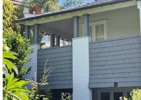
Figure 4.17 Detailed view of the balcony with rendered columns with timber accent, and timber shingles, looking northwest.
