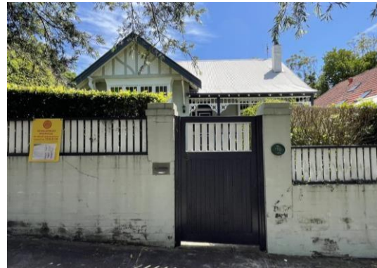
Figure 4.8 View of 119 Holt Avenue from the street, looking north.
