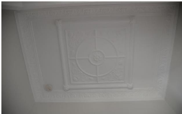
Figure 5.48 Ground floor apartment to east—east— original decorative plaster ceilings.
