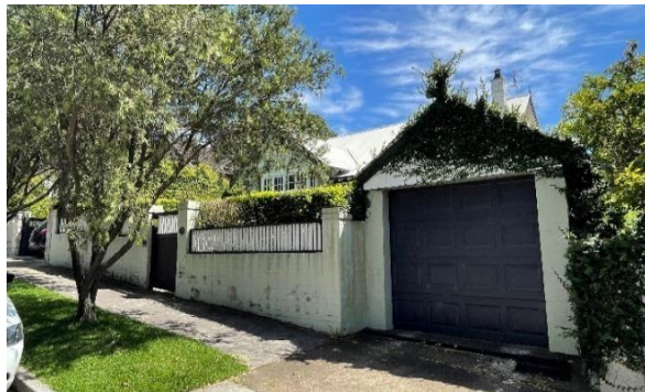
Figure 5.31 View showing the garage addition, looking northwest.
