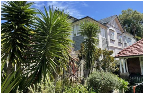
Figure 4.18 View showing a detail of the upper storey of the eastern elevation. The enclosed balcony, with timber detailing, is visible.
