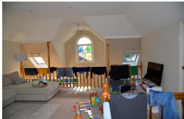
Figure 5.28 View of the attic floor fittings.
