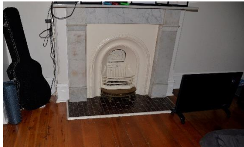
Figure 5.65 View of the original fireplace to the living room.
