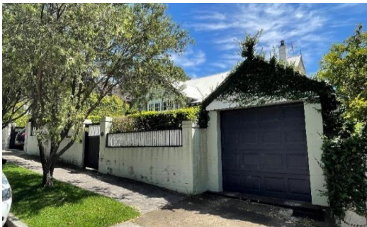
Figure 4.9 View showing the garage addition, looking northwest.
