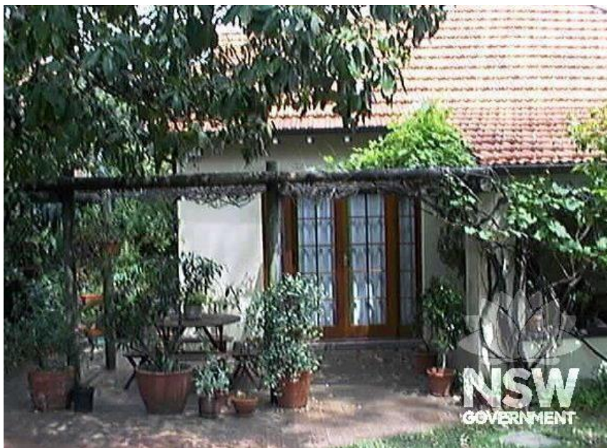
Figure 6.6 (Source: NSW State Heritage Inventory)
