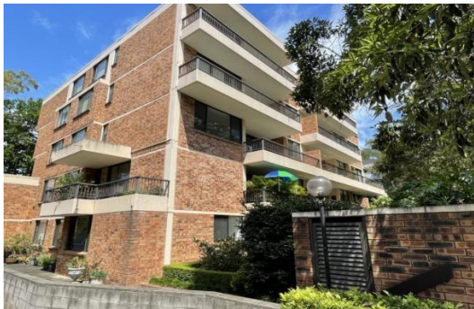
Figure 4.28 View of a typical contemporary apartment building.
