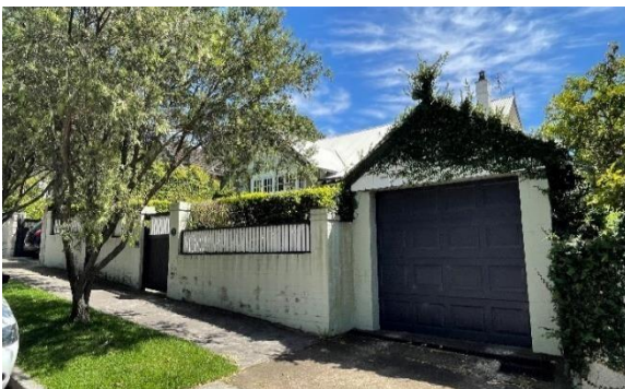
Figure 4.9 View showing the garage addition, looking northwest.
