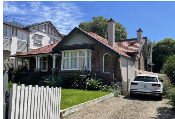
Figure 5.43 View showing the elevation, roof form and temporary car shade, looking northwest.
