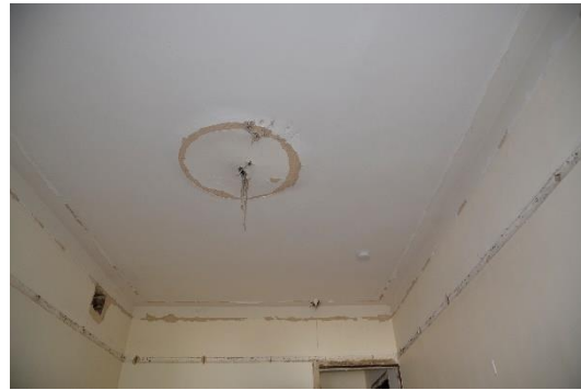
Figure 5.71 View of the ceiling to the front room with the ceiling rose and cornices
