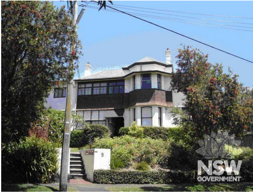
Figure 6.17 Primary façade of 'Dunbrody', 9 Davidson Parade. (Source: NSW State Heritage Inventory)
