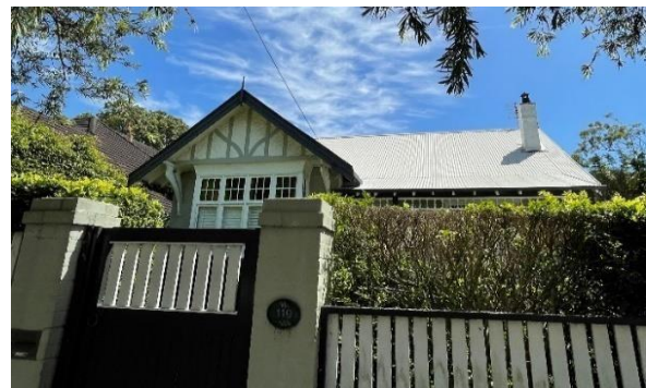
Figure 4.10 View showing a detail of the roof form, with decorative timber detailing, brackets and finial.
