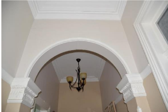
Figure 5.23 View of the hallway arch with plaster moulding.
