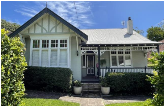
Figure 4.7 View of the primary elevation of 119 Holt Avenue.
