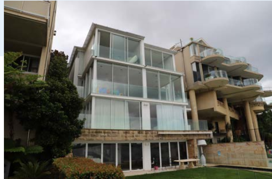
Photo. 13 Detail of south elevation at 3 Baden Road
