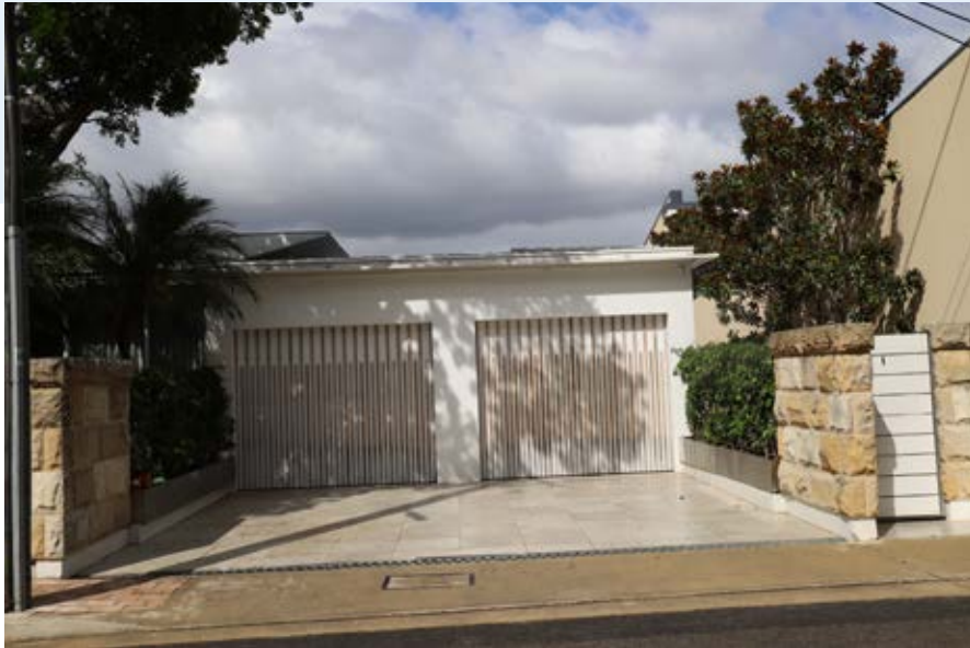
Photo. 18 Detail of 3-3a Baden Road Garage
