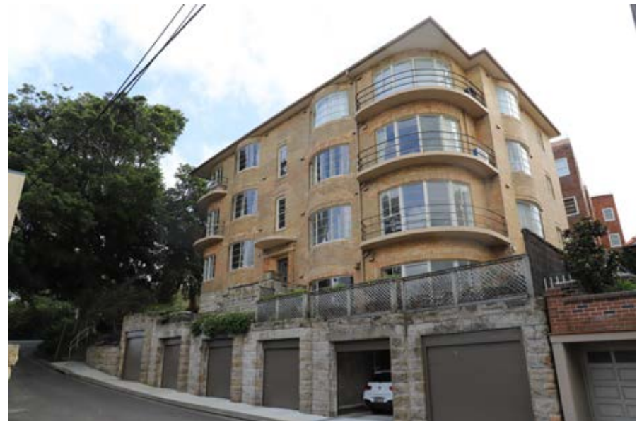
Photo. 15 Detail of the south and east elevation of 200 Kurraba Road
