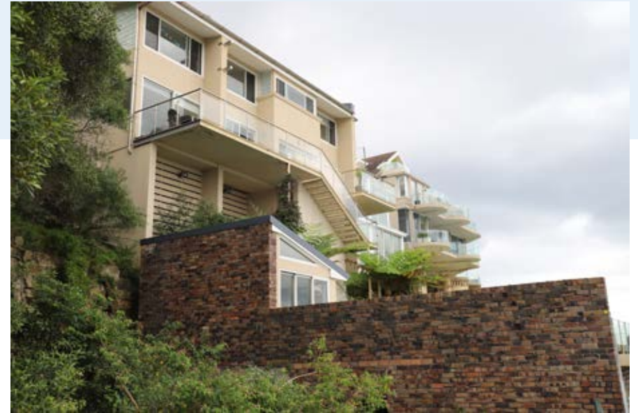
Photo. 5 Detail of south elevation of 1 Baden Road from the south-east edge of Kurraba Point Reserve
