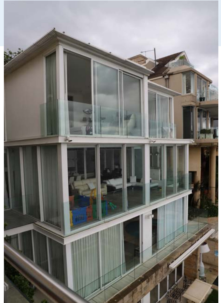
Photo. 11 Detail of south elevation of 3 Baden Road from an external balcony at 1 Baden Road
