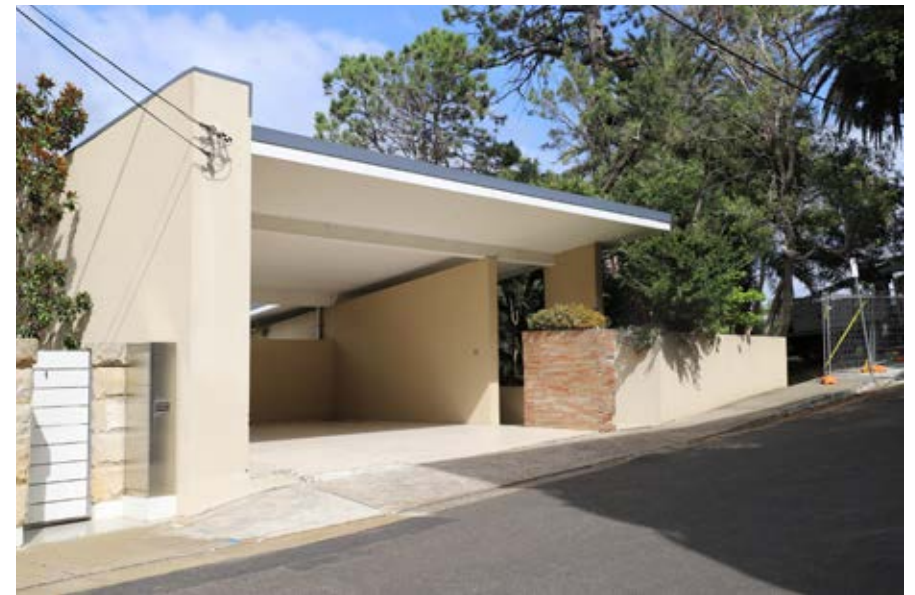
Photo. 17 Existing carport entry and roof form at 1 Baden Road
