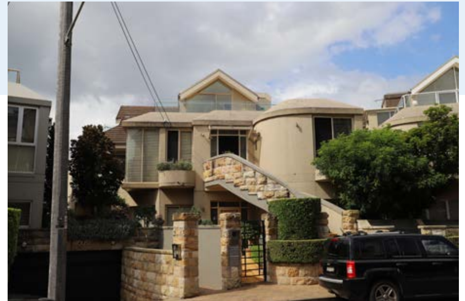
Photo. 22 Detail view of 9 Baden Road
