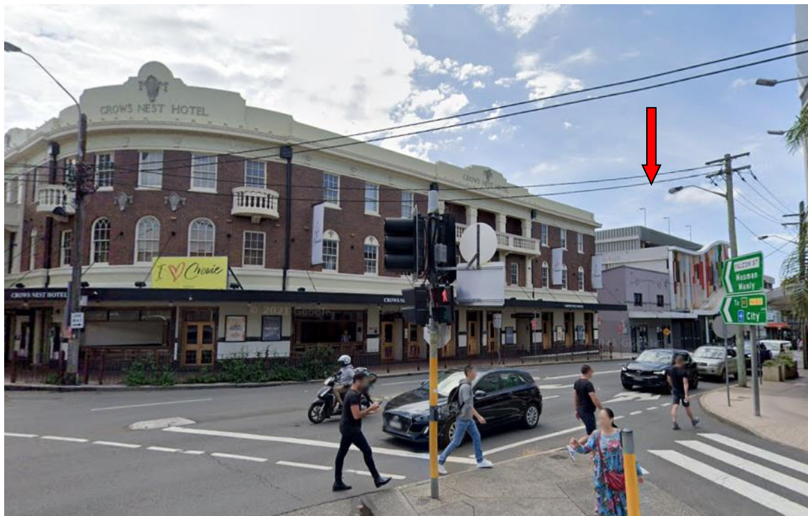
Figure 6 Heritage Listed 'Crows Nest Hotel' with Alexander Street carpark in the background (Source Google Maps)
