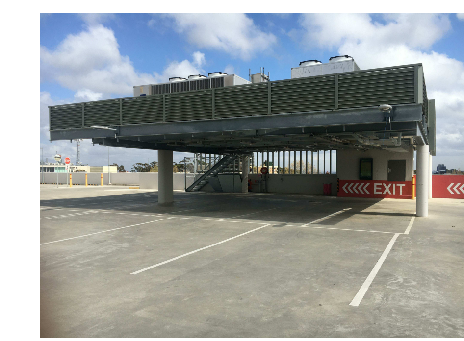
SITE PHOTO - ROOF PLANT STRUCTURE
