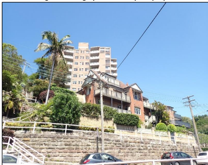
Figure 18. View looking west towards the subject site from the public footpath on the lower section of the Ellis Lookout Reserve. This currently open view of the projecting gable end of the original 1911 dwelling will be largely obscured by the proposed deck extension
