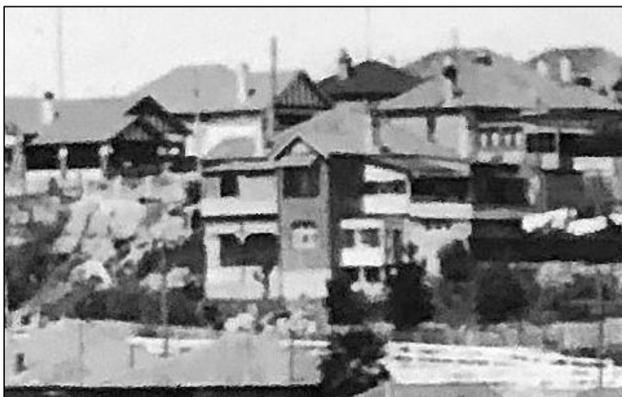
Figure 20. A close-up view of No. 80 Cairo Street from a 1939 photograph, showing the extent of the original balconies, which were partially enclosed with a roof on the ground floor level, and inset behind the eastern gable end of the dwelling. Source: Garibaldi Tyler (1939) – ‘Long Gully Bridge, Cammeray’ https://www.flickr.com/photos/183133849@N08/50257808758/
