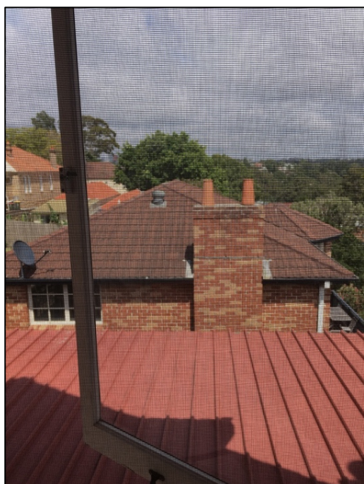
Photo 1: View over existing roof of No 32D Pine Street
