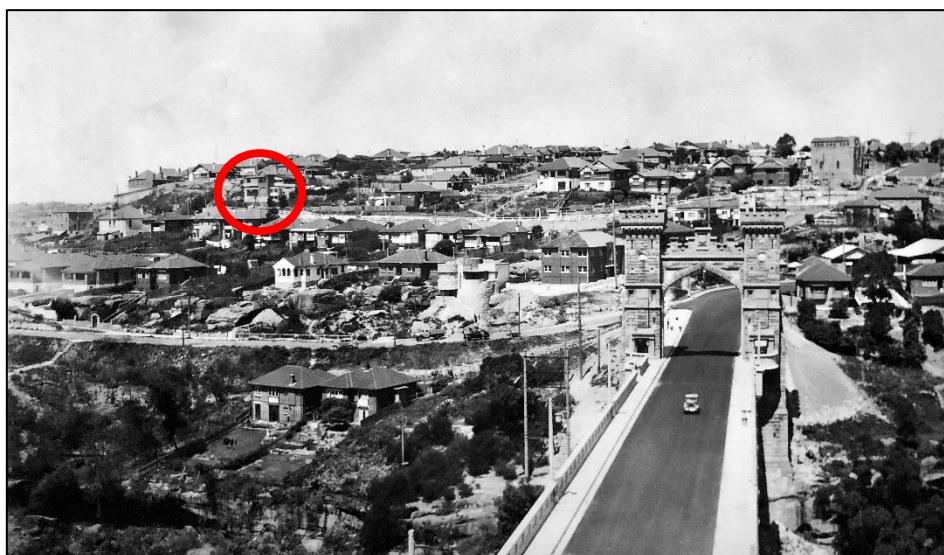
Figure 21. A 1939 photograph of the northern slopes of Cammeray and the Long Gully Bridge, with No. 80 Cairo Street shown by the red circle. Source: Garibaldi Tyler (1939) – ‘Long Gully Bridge, Cammeray’ https://www.flickr.com/photos/183133849@N08/50257808758/
