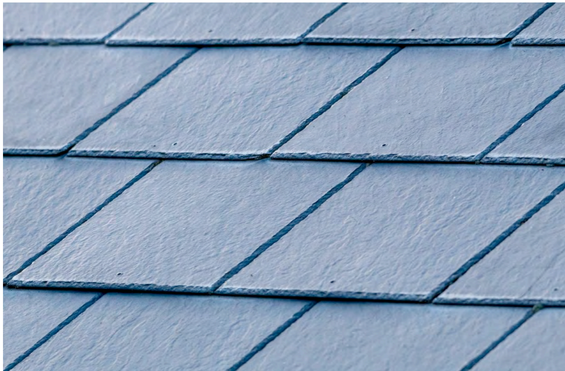
1. Slate like roof tiles
