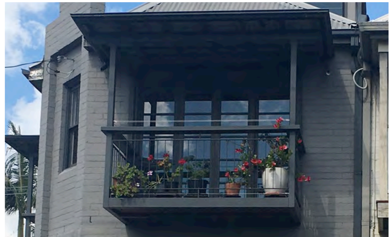
4. Open metal balustrading to existing attic balcony and new side deck
