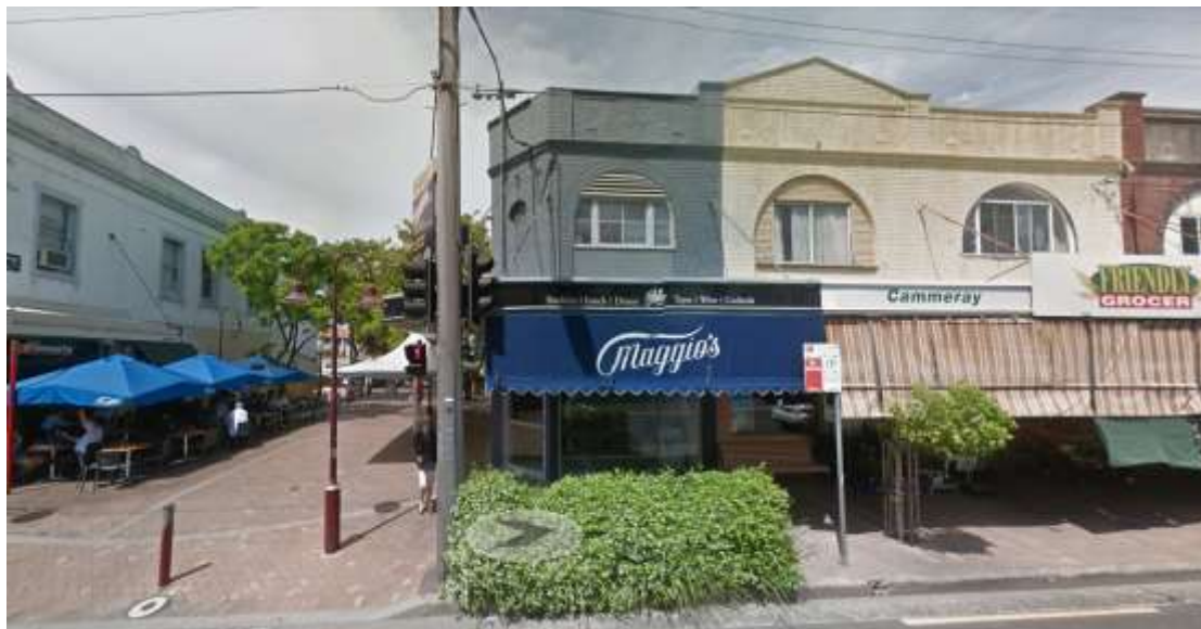
Figure 1: Front West Elevation to Miller Street. Subject property has the blue awning. [Source: Google Maps]
