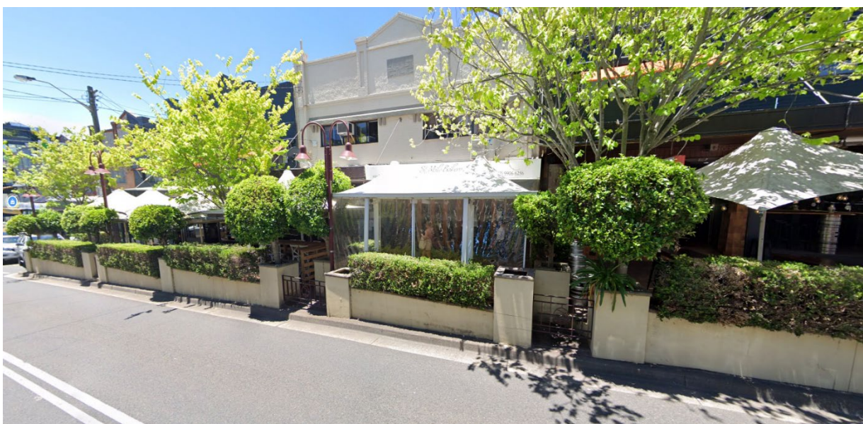
Figure 3 – Existing shadowing structures located along Willoughby Road
