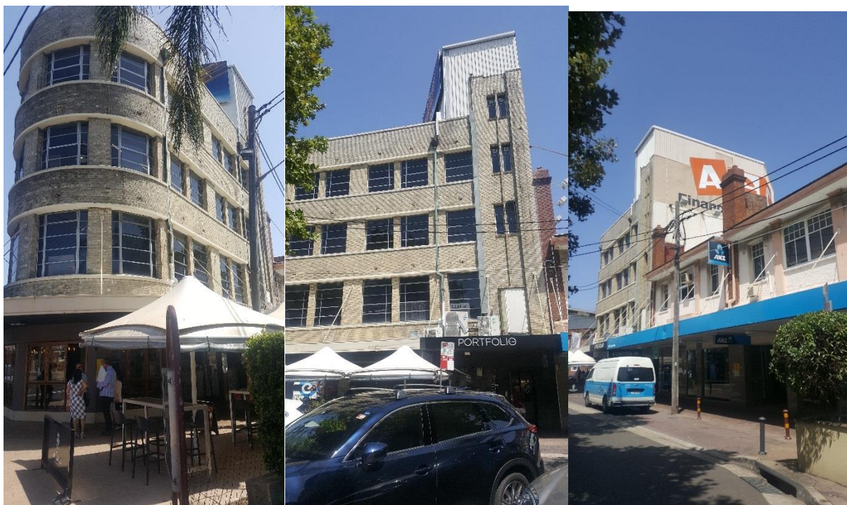
Figures 4, 5 and 6 – Existing building on the subject site – southern (left), eastern (middle) and northern (right) elevations of the building
