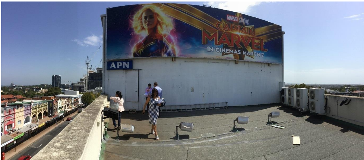
Figure 7 – Southern elevation of the metal clad structure on the roof of the northern part of the building
