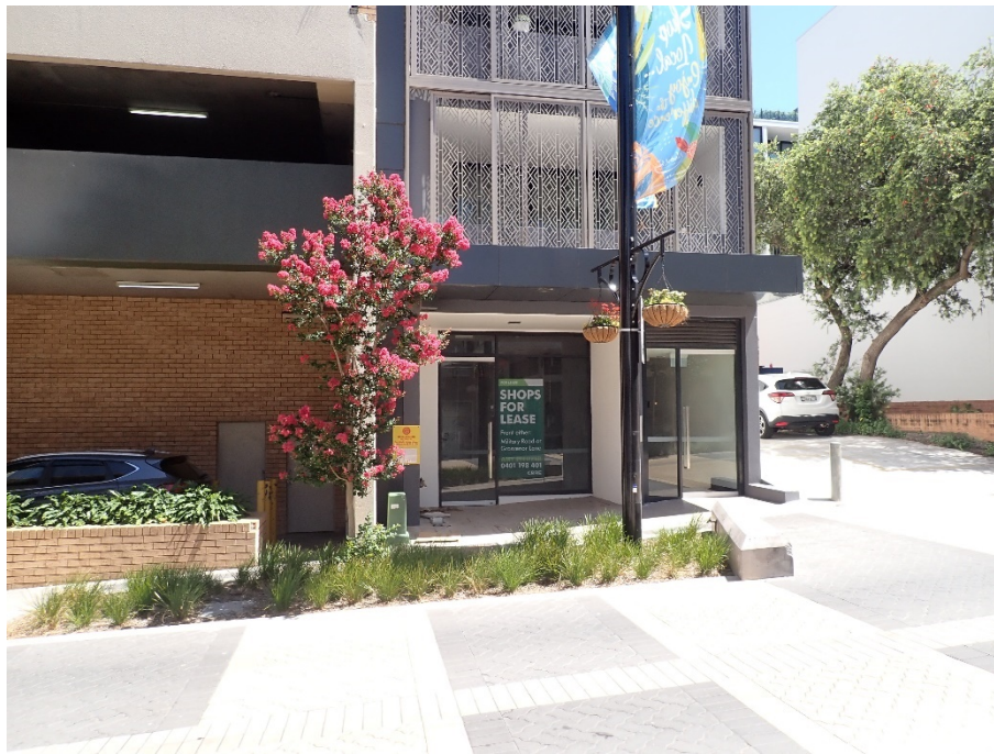
Figure 5. Site Photo of Grosvenor Laneway including the public domain upgrade works.
