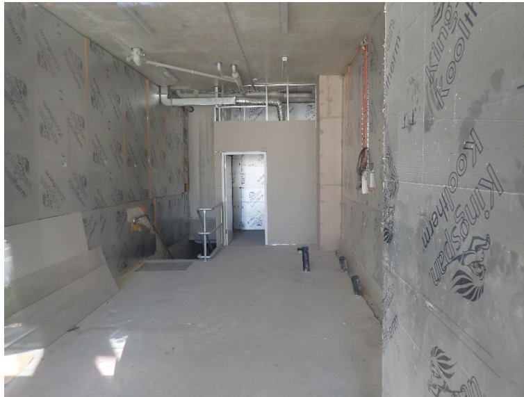
Figure 7. Site photo of the ground floor of the cold shell tenancy
