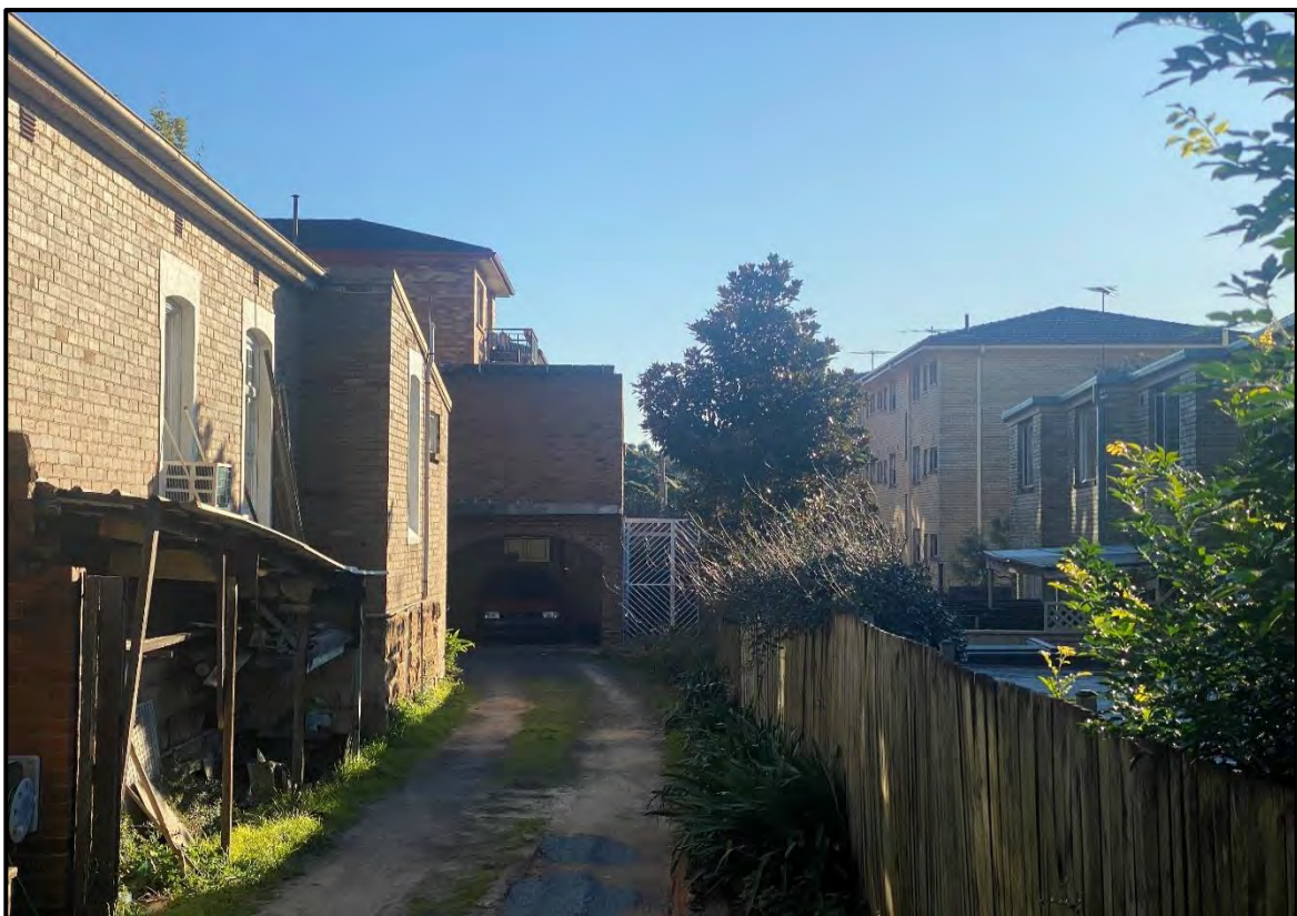
Figure 21: Rear (western) – Willoughby Lane elevation of properties at No. 82 and 84 Alexander Street
