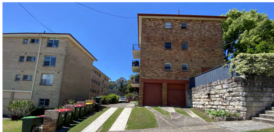
03 - Abbott Street footpath, looking east towards site between adjacent buildings
