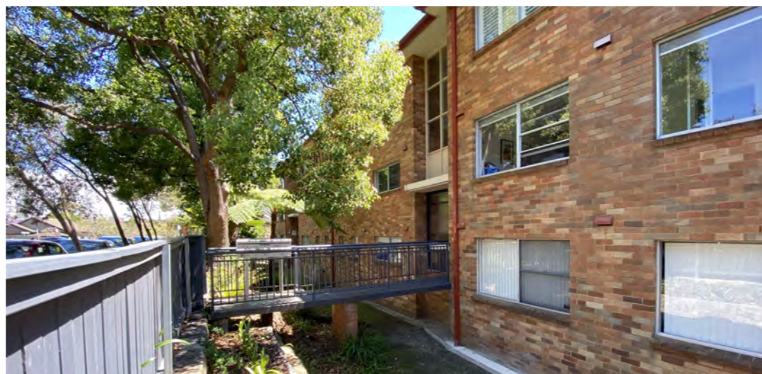
04 - Vale Street footpath, looking west along adjacent property's street boundary
