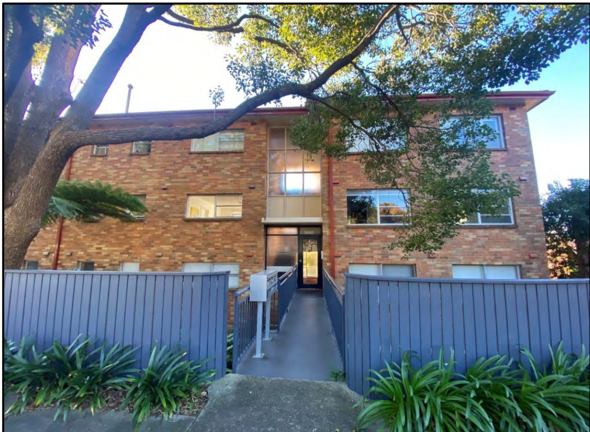
Figure 28: Residential flat building at No. 49 Abbott Street
