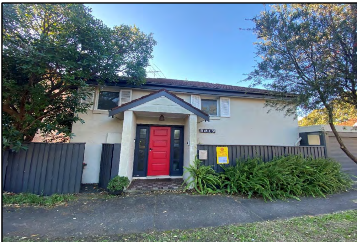
Figure 19: Front of dwelling house at No. 18 Vale Street
