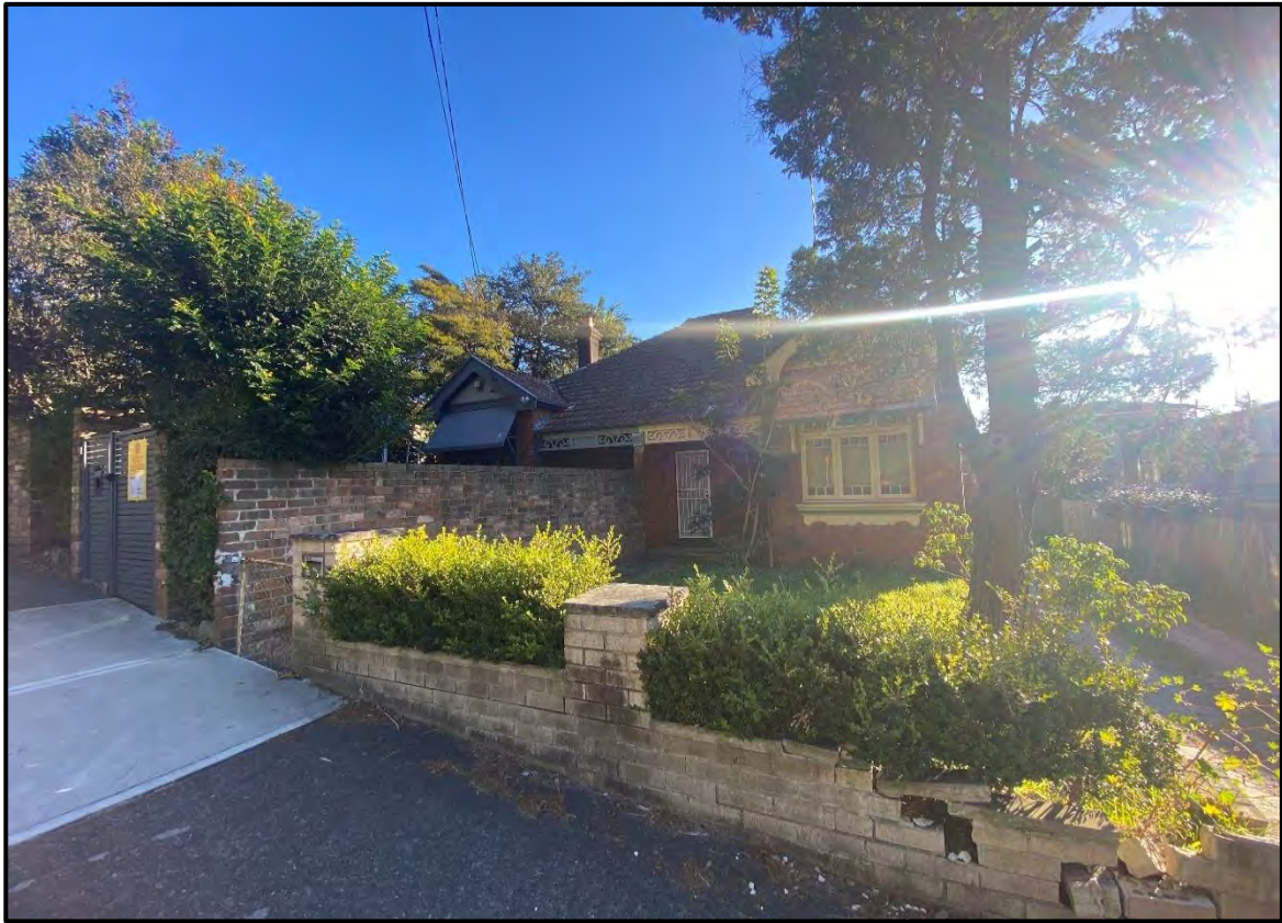
Figure 20: Front of properties (semi-detached dwellings) at No. 560-562 Miller Street
