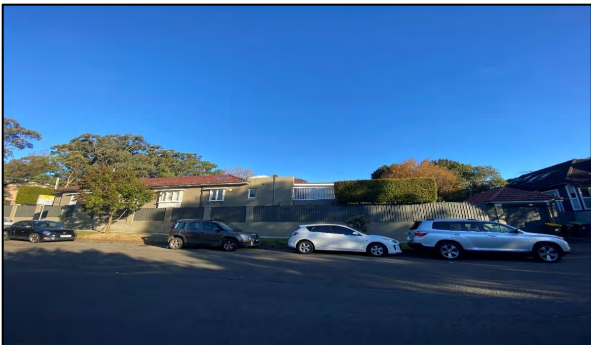
Figure 26: Dwelling house at No. 556 Miller Street
