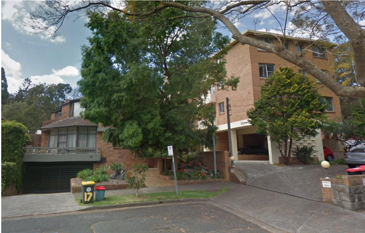
Figure 2J – Residential flat buildings on Priory Road
