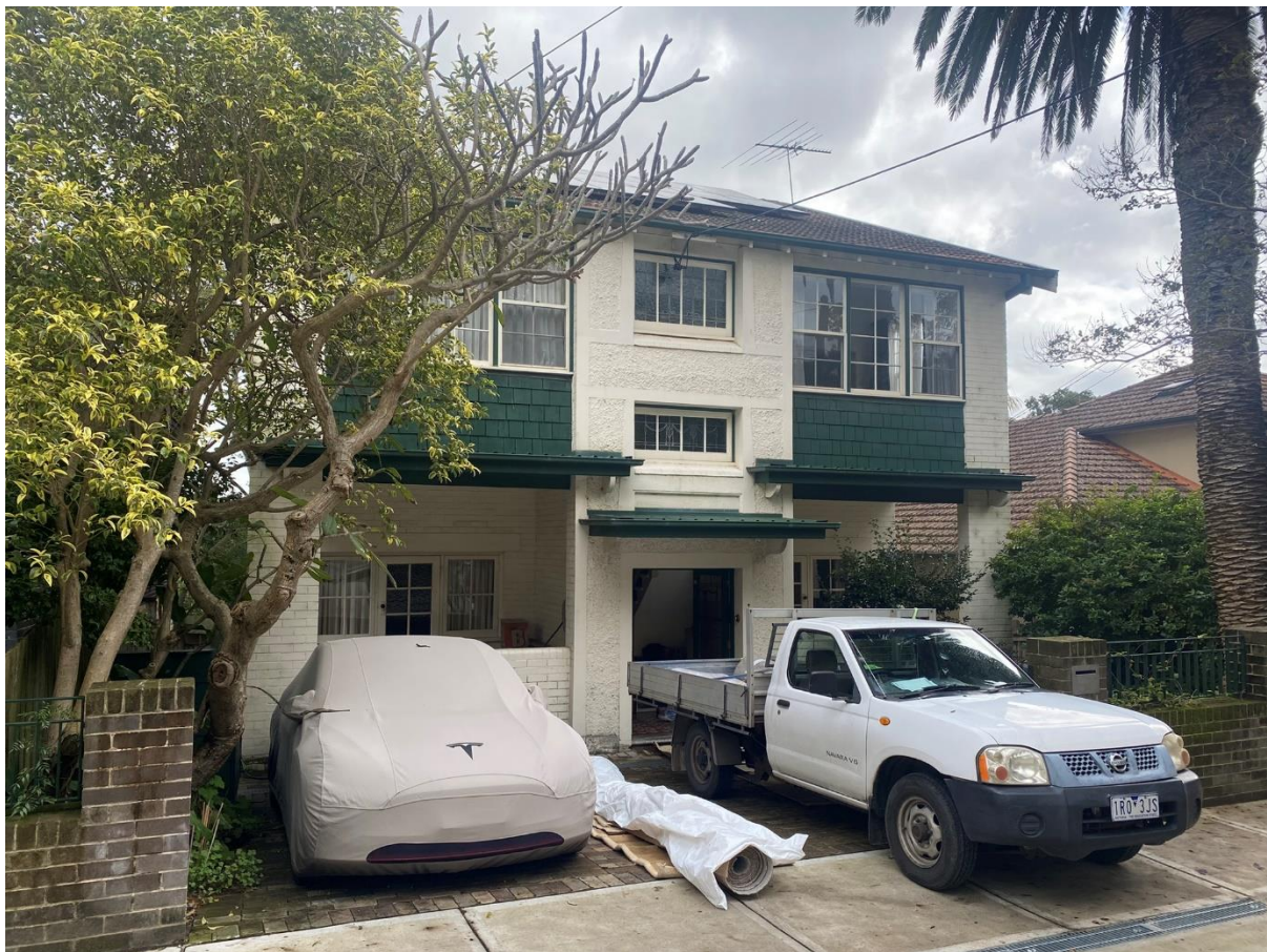
Figure 2G – No. 50 Edward Street (north of the subject site)
