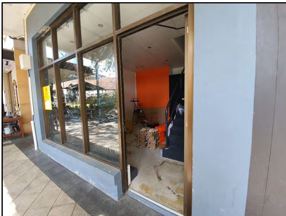
Figure 9: View into the internal area of subject site at ground level
