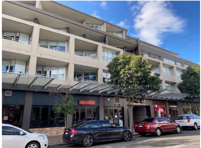
Figure 16 Development on the eastern side of Rangers Road
