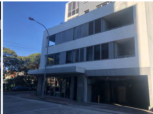
Figure 18 Development on the eastern side of Rangers Road
