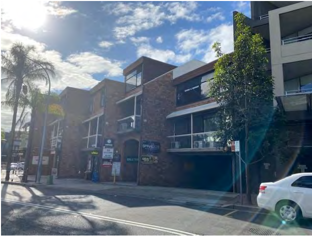
Figure 15 Development on the eastern side of Rangers Road
