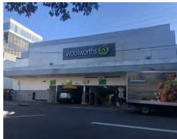
FIGURE 8: Existing Woolworths underground carpark entry (Yeo Street)
