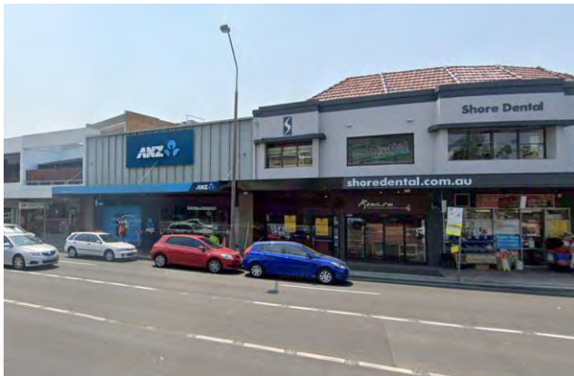
Figure 11 Development on the northern side of Military Road
