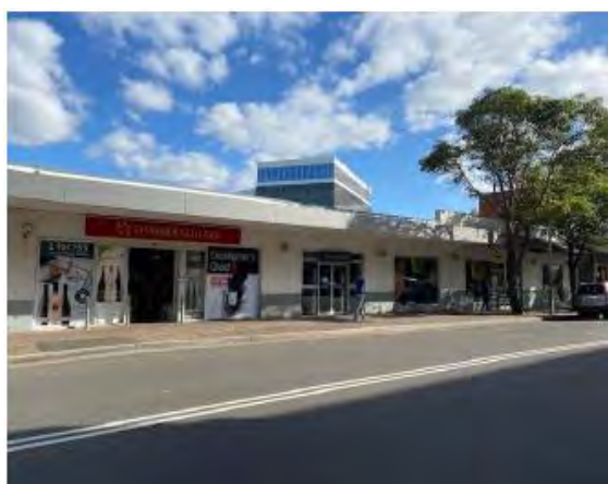
FIGURE 7: Existing Woolworths (1-7 Rangers Road)
