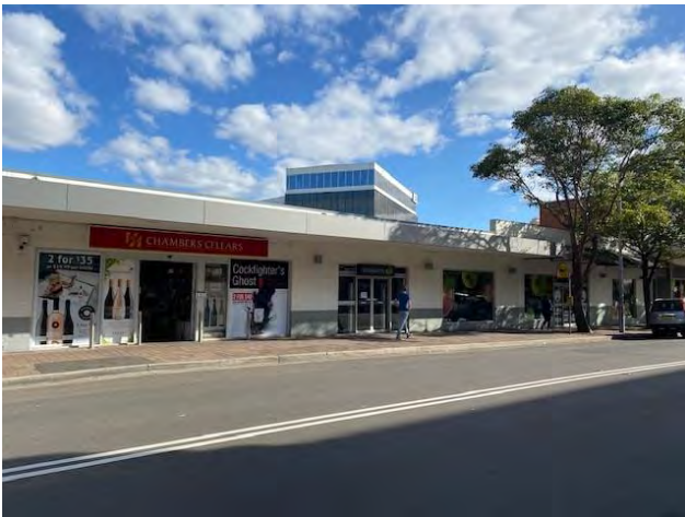
Figure 7 Existing Woolworths and bottle shop
