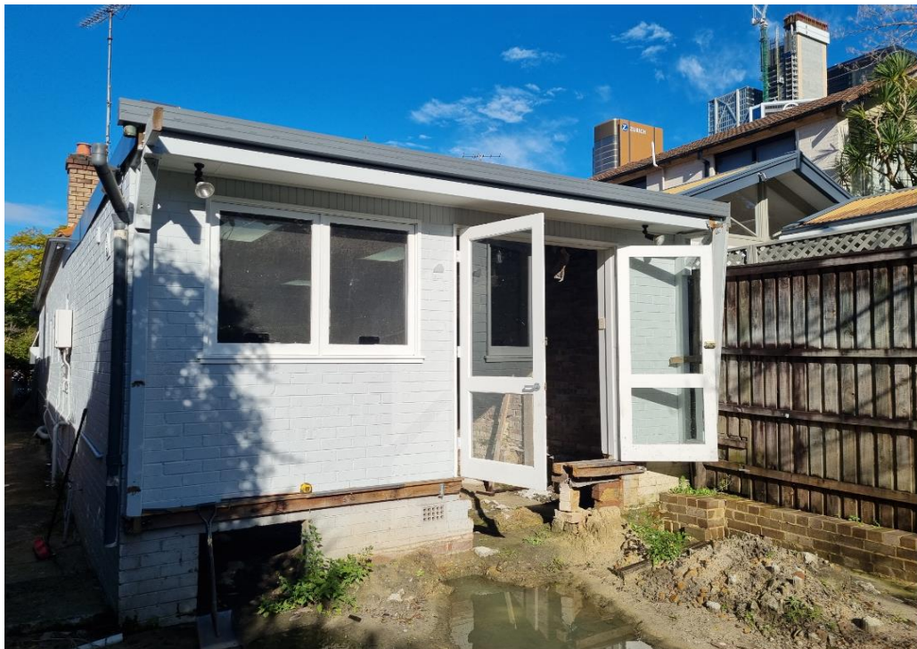
Figure 9: Subject site (rear elevation) Site Visit
