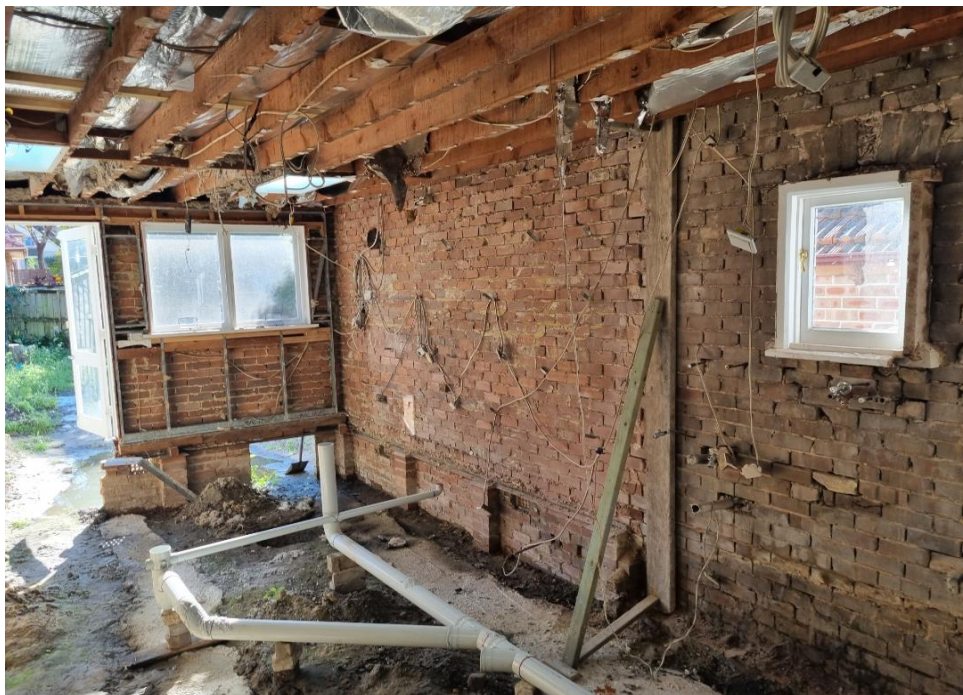
Figure 10: Subject site (internal rear addition) Site Visit
