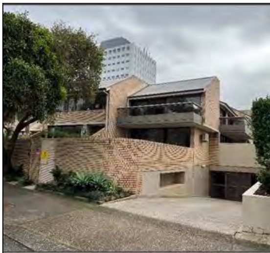
Figure 7 View of the rear of the subject site, showing the existing balcony structure
