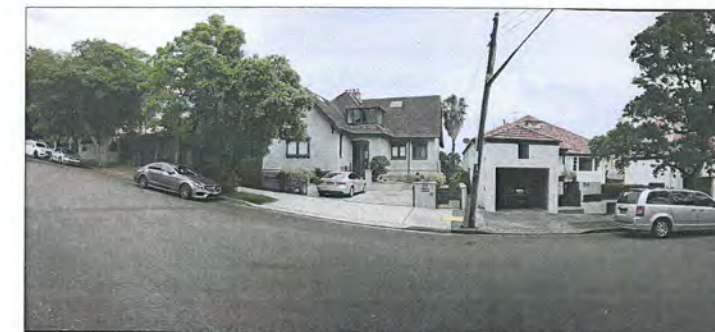
SUBJECT SITE - EXISTING STREET VIEW
