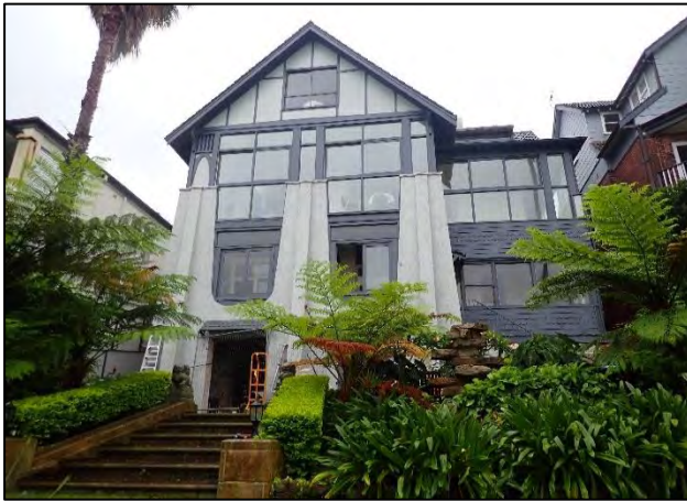
Figure 10. View of the southern elevation from the rear garden.
