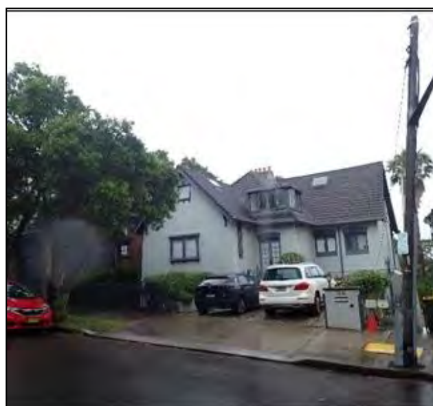
Figure 4. View of the site from Lower Wycombe Road.
