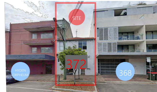
STREET VIEW ALONG PARRAWEEN STREET
