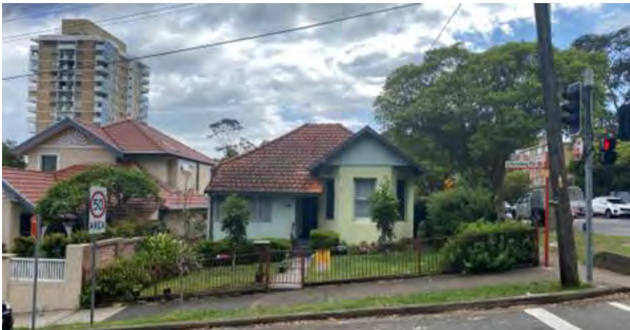
Existing Benelong Road elevation
