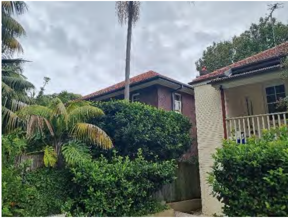
Figure 24. No. 7 Undercliff Street from the rear of the subject site
