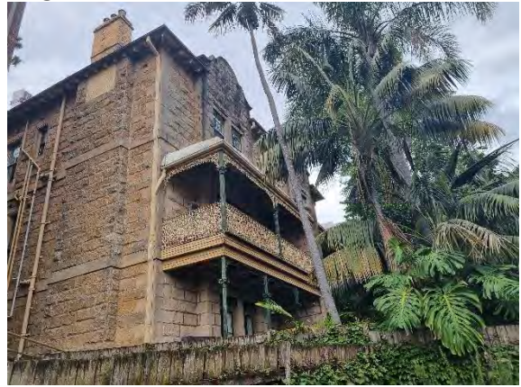
Figure 25. No. 5 Harriatte Street from the rear of the subject site
