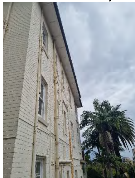
Figure 33. Northwestern elevation of the existing building
