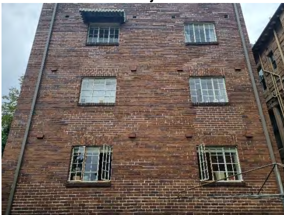
Figure 26. No. 1 Harriette Street from the rear of the subject site
