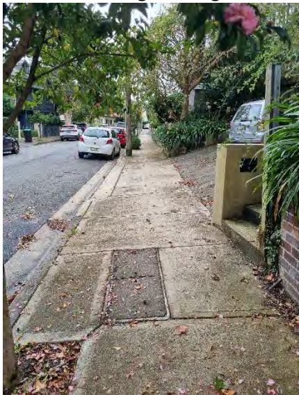
Figure 14. Undercliff Street footpath
