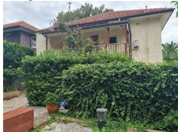
Figure 19. Rear of the existing building
