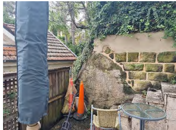
Figure 21. Retaining wall and rocky outcrop adjacent to No. 23 Undercliff Street
