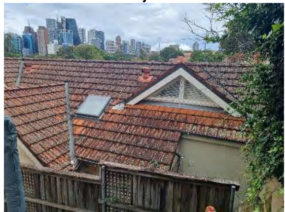
Figure 27. No. 23 Undercliff Street from the rear of the subject site
