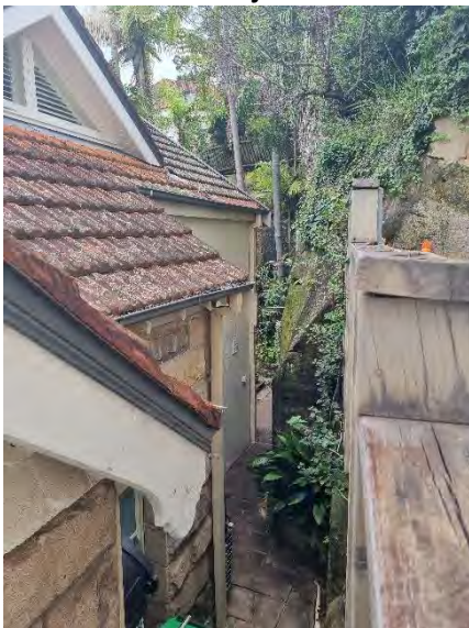
Figure 30. Southeastern side of No. 23 Undercliff Street
