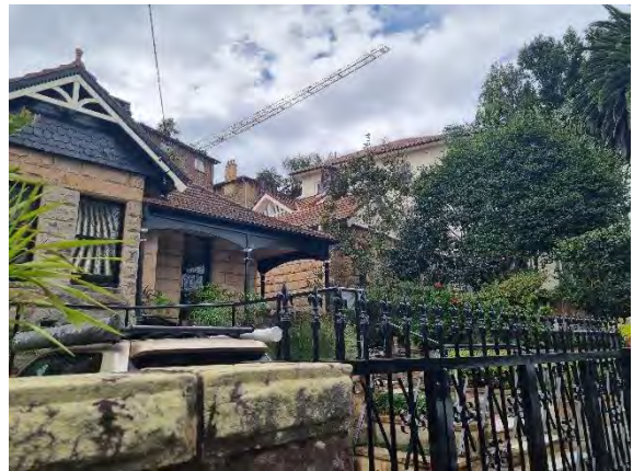
Figure 13. Nos. 25 & 23 Undercliff Street
