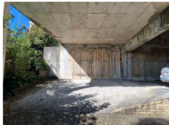
Figure 27. Existing excavated parking area
