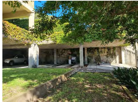
Figure 25. Existing excavated parking area
