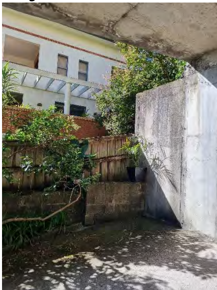
Figure 32. No. 8 Sutherland from southern end of existing driveway
