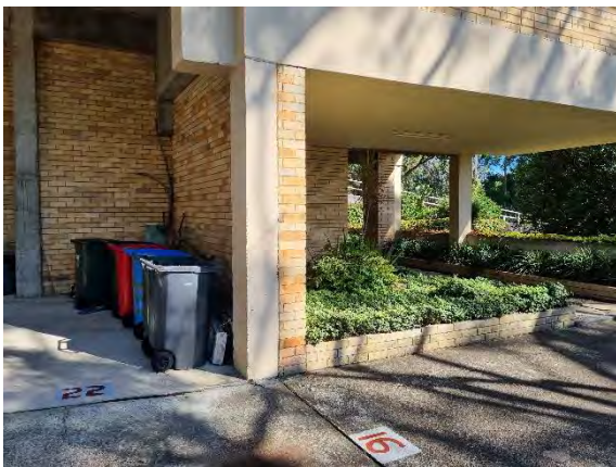
Figure 26. Existing excavated parking and undercroft area
