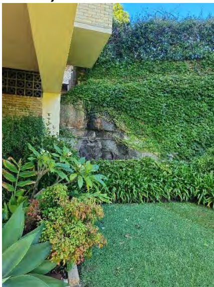
Figure 22. Existing western side undercroft and courtyard below Park Avenue
