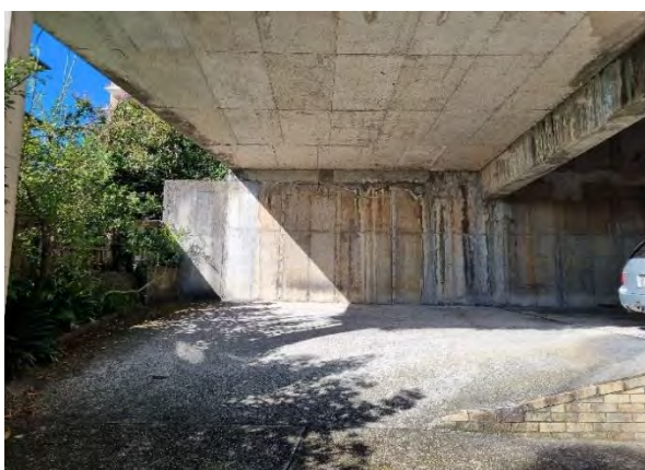
Figure 47. Existing retaining wall adjacent to the eastern side boundary
