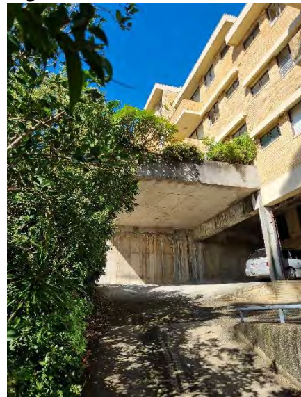
Figure 33. Eastern side of existing building
