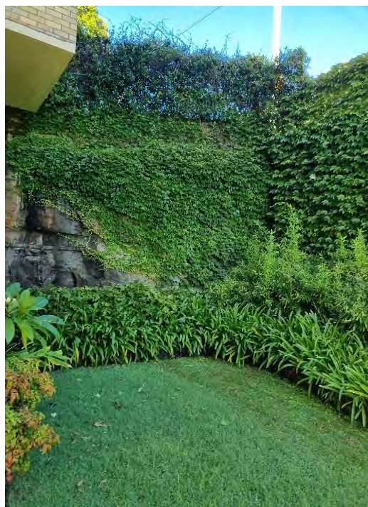
Figure 58. Site photo of existing land levels within the eastern side setback adjacent to Park Avenue
