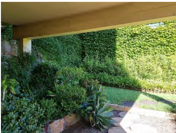
Figure 20. Existing western side undercroft and courtyard below Park Avenue
