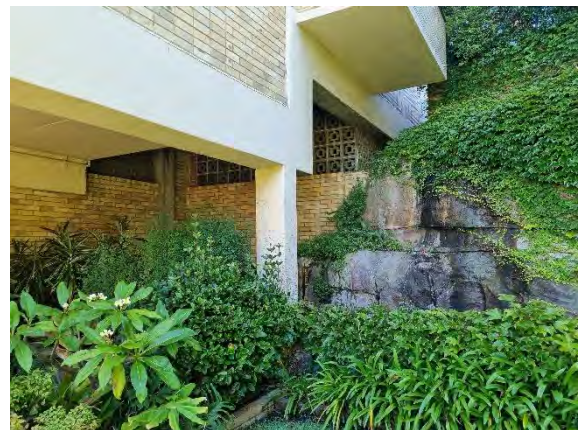
Figure 21. Existing western side undercroft and courtyard below Park Avenue
