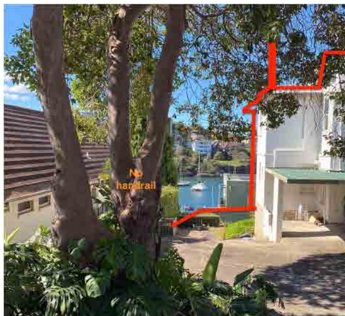
View from deck of 170 Kurraba Road showing impact of the revised DA scheme. Handrail is not required because of changes to retaining wall and garden design.
