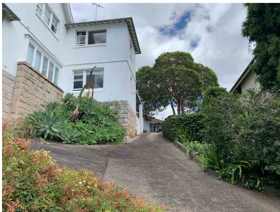
View to the west of paved north garden showing change in levels and 170 Kurraba Road behind with water views through the northern setback.
