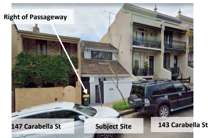
Figure 8: Subject site (Carabella Street Elevation)
