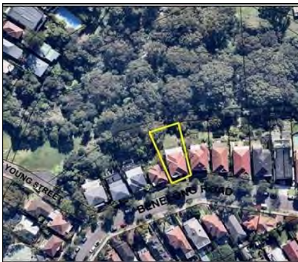
Figure 5. Aerial photograph of subject site (outlined yellow) and surrounding development
