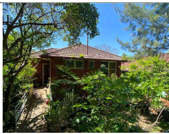
Figure 5: The front elevation of the dwelling
