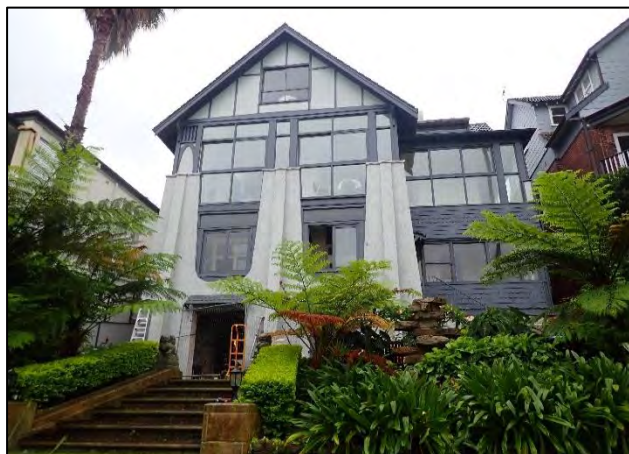
Figure 10. View of the southern elevation from the rear garden.
