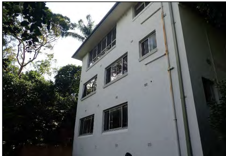
Figure 10. Western rear view of the existing building.
