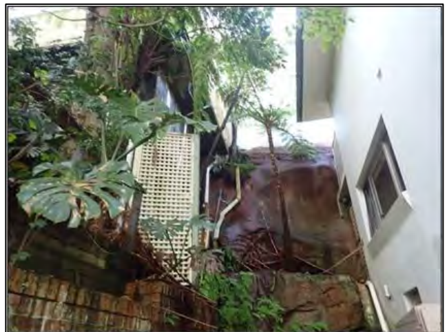
Figure 9. View of the northern side setback with 20 Tobruk Avenue (left) towards the garage.
