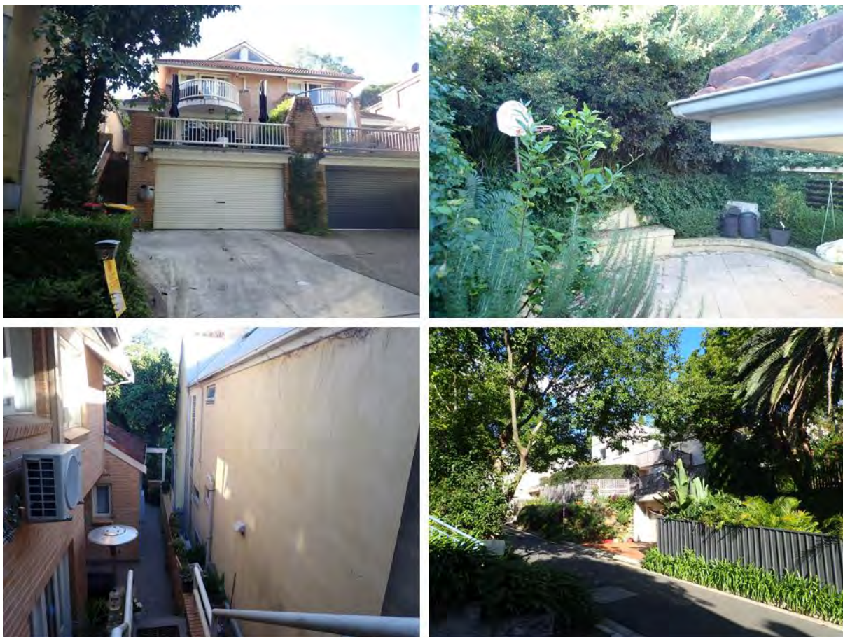
Figure 3 – Subject Site Front Elevation and rear garden (top) and side setback and landscaping within Carlyle Lane (below)
