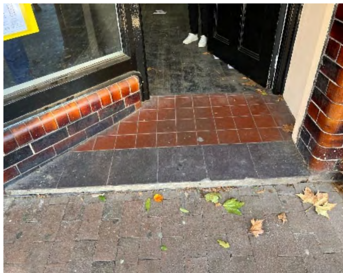
Figure 15: Threshold entry from Miller Street
