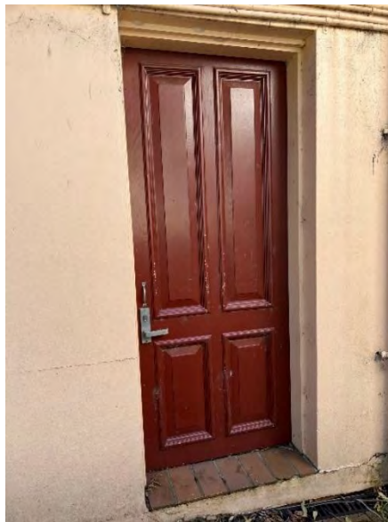
Figure 16: Replacement of Existing Period Door
