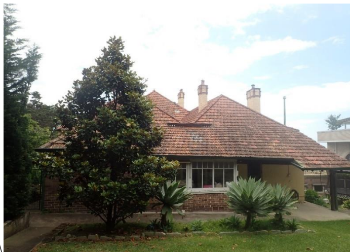
Figure 8: Subject site (Rear elevation)
