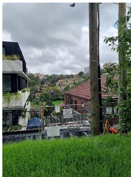
Figure 15. Site Photo of No. 20 Premier Street and the Subject Site
