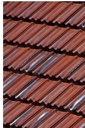
9 TERRACOTTA TILED ROOF
