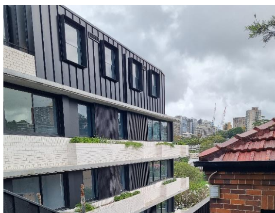
Figure 21. Northern elevation of adjoining residential flat building (No. 20 Premier Street)
