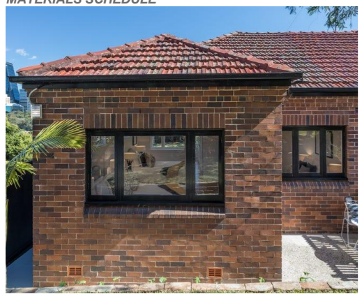
1 EXISTING BRICKWORK AND TERRACOTTA ROOF
