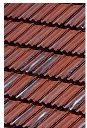
9 TERRACOTTA TILED ROOF
