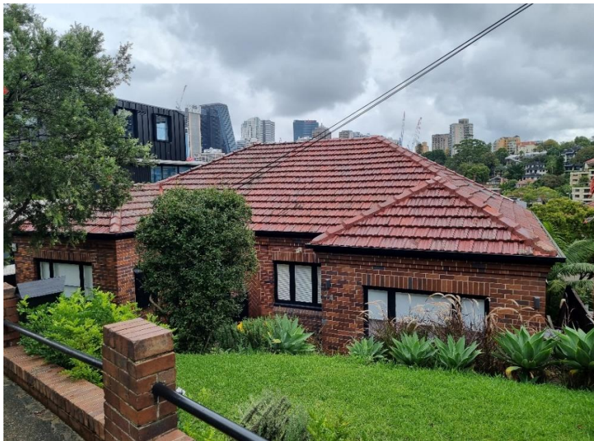
Figure 9. Site photo of pair of existing semi-detached dwellings.
