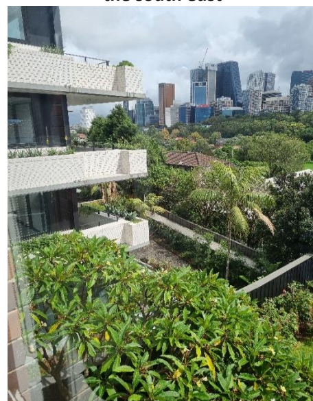
Figure 13. Site photo of rear of the RFB at No. 20 Premier Street
