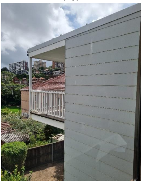
Figure 12. Site photo of rear addition of No. 24 Premier Street
