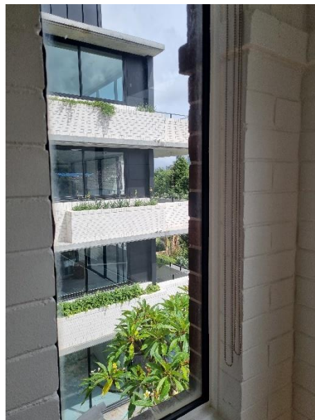
Figure 25. Northern elevation of adjoining residential flat building
