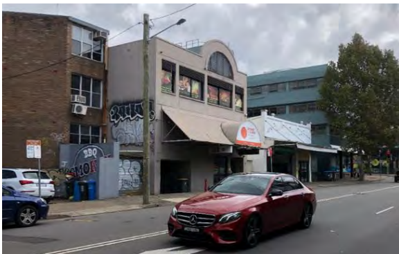
Figure 8: View of northern end of eastern frontage (Alexander Street)
