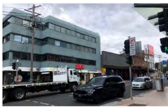
FIGURE 9: View of north-eastern frontage (Falcon Street)
