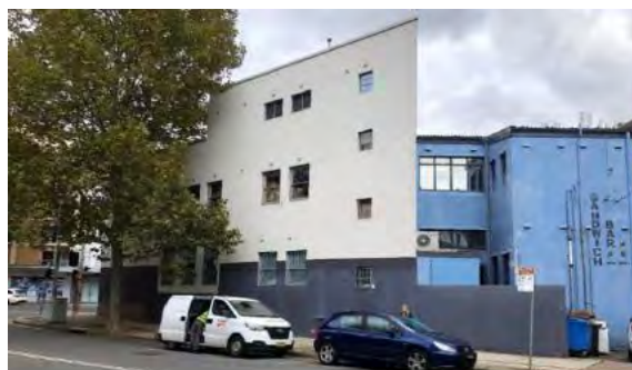
FIGURE 7: View of south-eastern frontage (Alexander Street)
