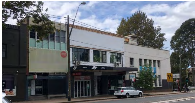
Figure 13: View of southern end of western frontage (Pacific Highway)
