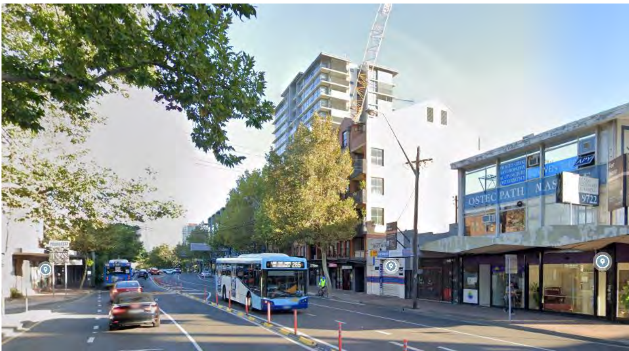
Figure 17: Development at 210-220 Pacific Highway (Source: Google Maps)
