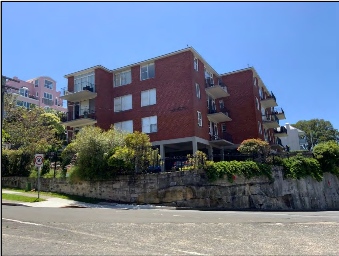
Figure 26: Western and south-western sides of existing building and rock wall – viewed from Blues Point Road
