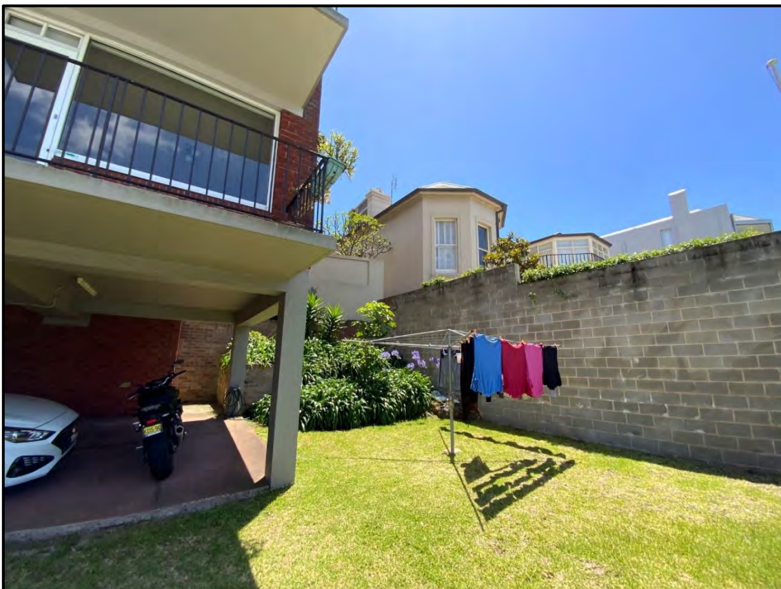
Figure 31: Undercover parking, clothes drying area and landscaping and rear view of No. 3 Warung Street
