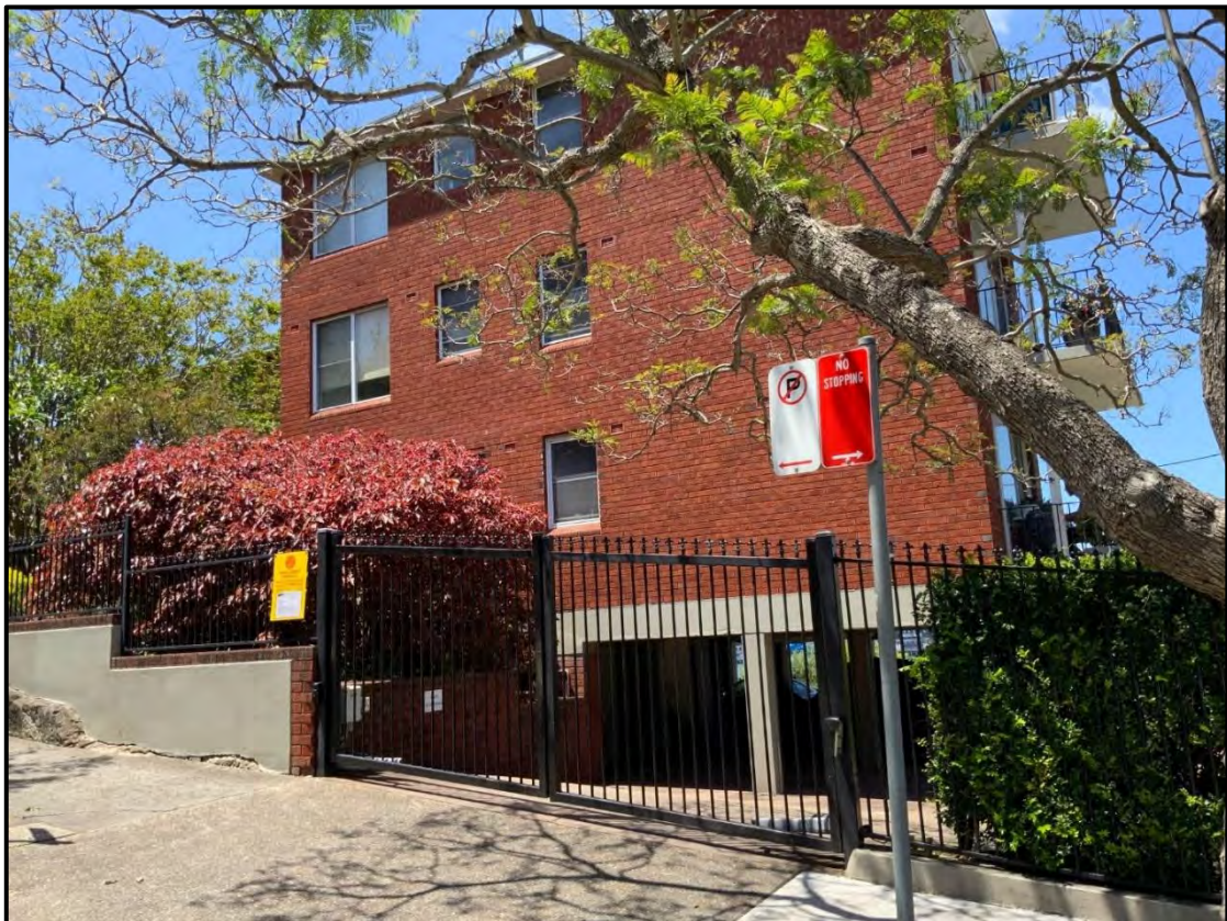
Figure 23: Front driveway of existing residential flat building – viewed from Warung Street
