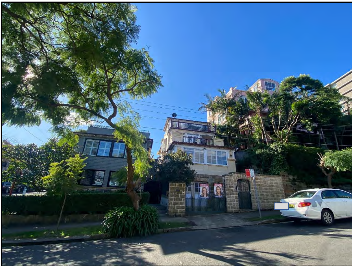
Figure 33: Front of residences at No.'s 2, 4 and 6 Warung Street
