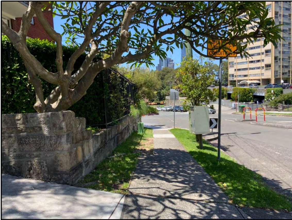
Figure 32: Rock wall along western boundary of site
