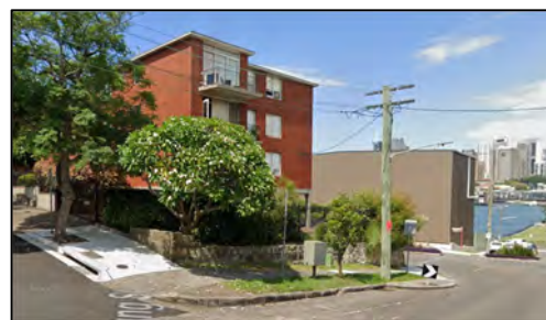
Figure 10b: View from Blues Point Road across western façade of building
