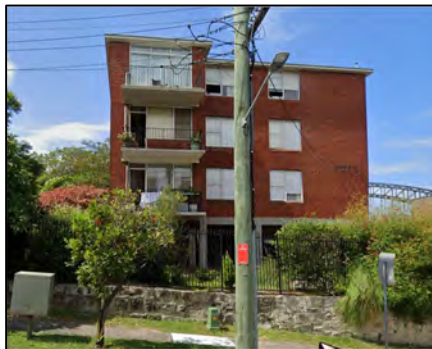
Figure 8: Existing western façade
