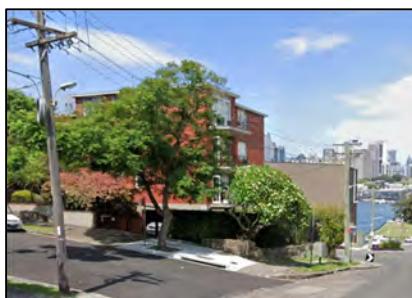
Figure 10a: View from Blues Point Road across western façade of building
