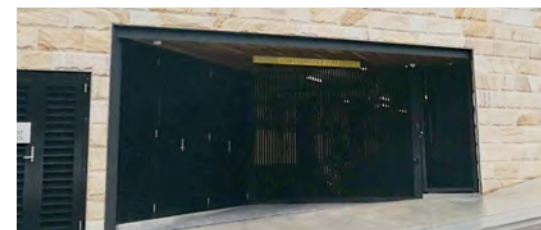
C. BASEMENT GATE. DARK GREY PAINTED METAL 20 x 20mm SHS @ 40mm CENTRES
