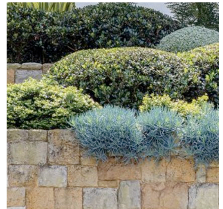
RETAINING WALL SANDSTONE
