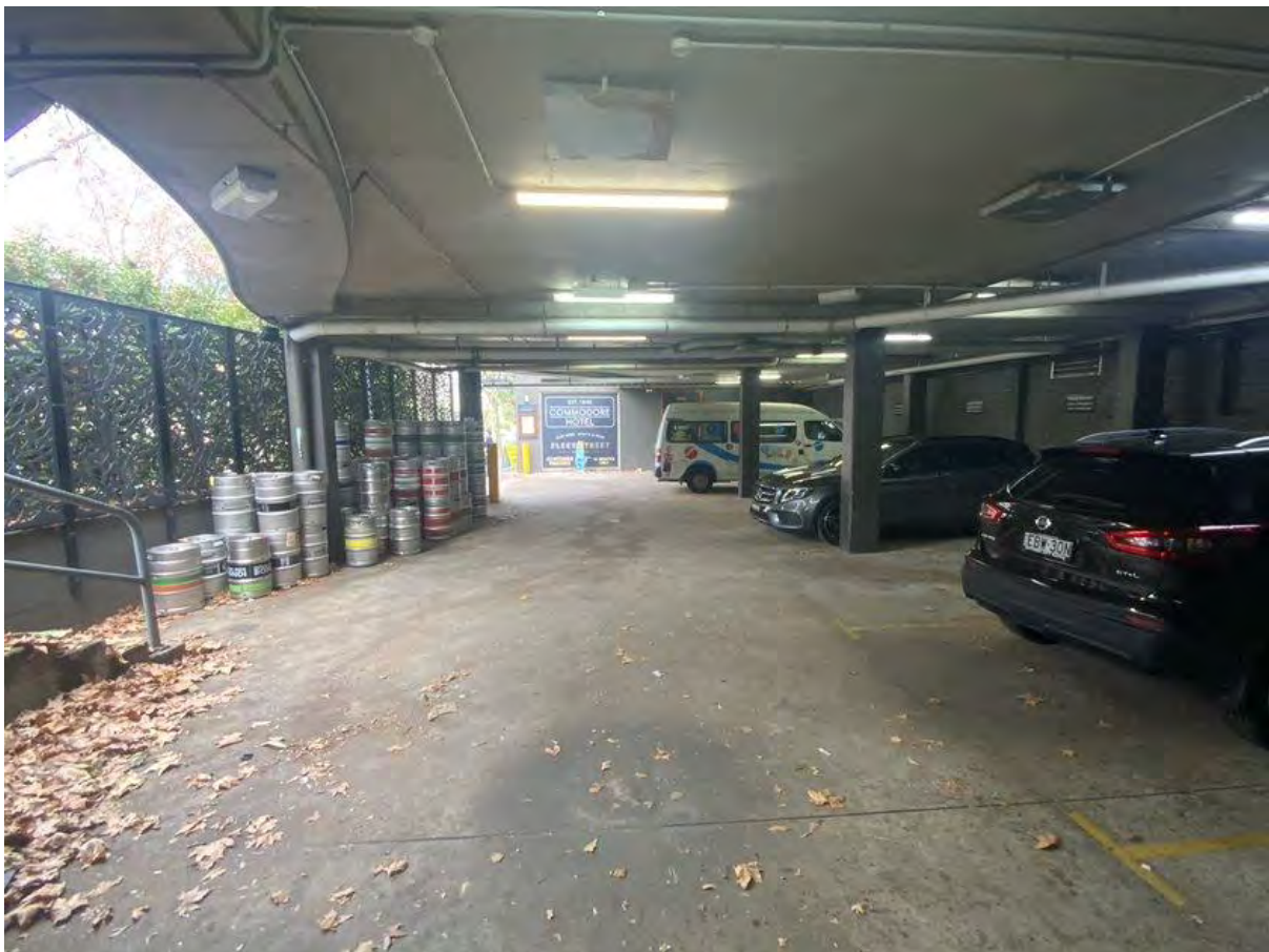
Figure 5 – Existing lower ground Car Park
