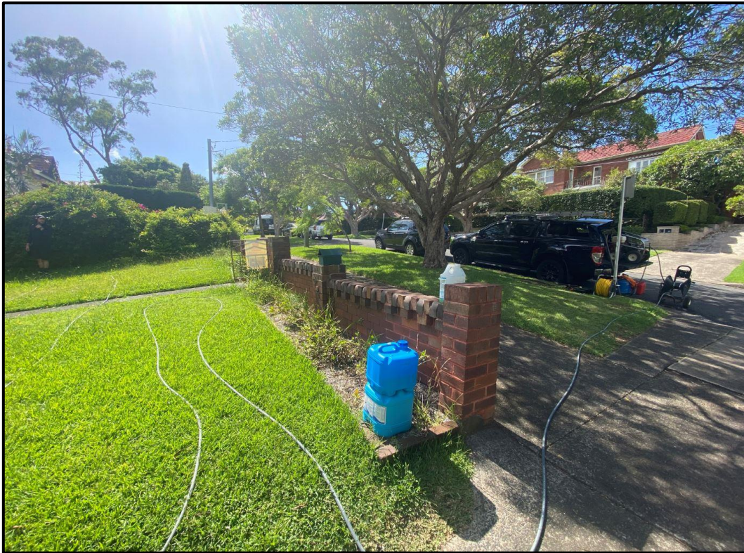
Figure 21: Existing front fence.
