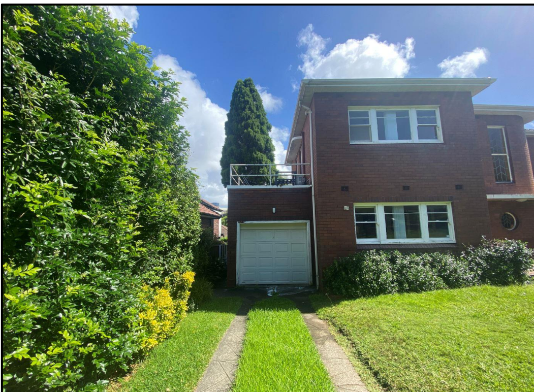
Figure 14: Front of dwelling and attached garage with roof terrace.
