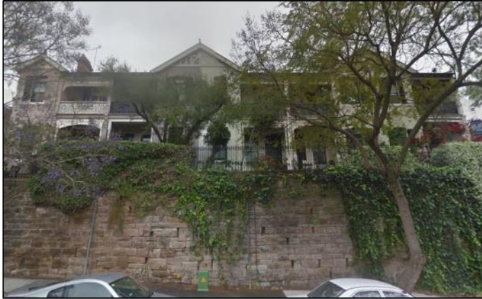
Figure 22: Nos. 100-108 Carabella Street, the terrace house group, of which the subject site forms part. Google Maps.
