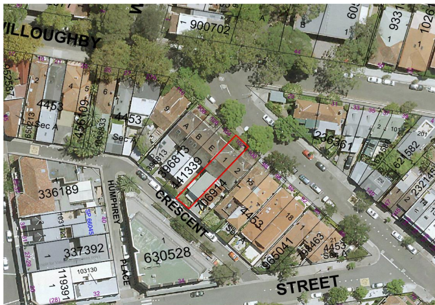
Figure 4 - Aerial Photo of site (edged in red) and surrounds (North Sydney Council, 2018)
