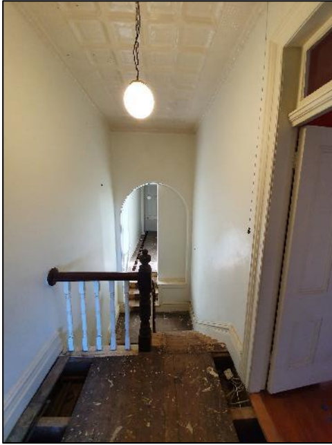
Figure 14: Stair hall, view looking south west. GVP Design Studio.
