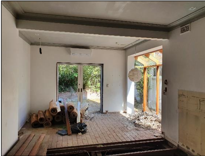
Figure 12: Sun room, looking south west. GVP Design Studio.
