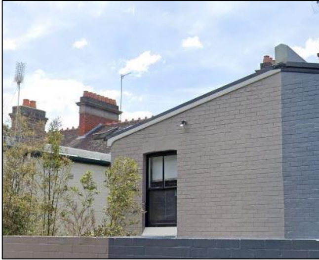
Figure 10: Detail of the south western (rear) elevation at first floor level.
