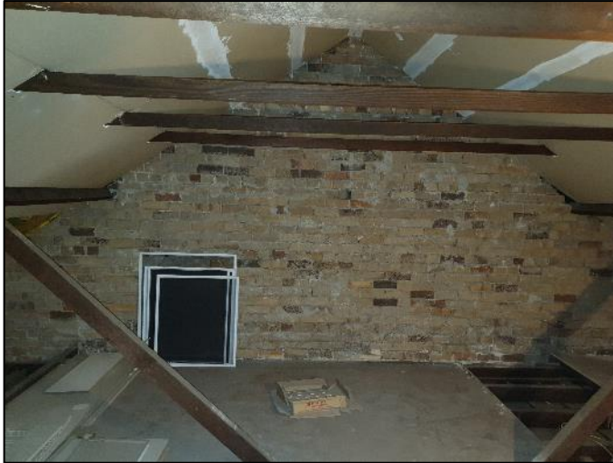
Figure 18: Attic, looking south east. GVP Design Studio.
